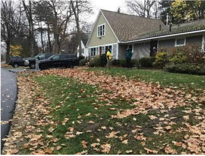
View of 86 Walker Bungalow Road and front yard from the road facing South.
