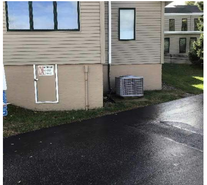
View of the entrance to the crawlspace and air conditioning unit to the right standing in the North
