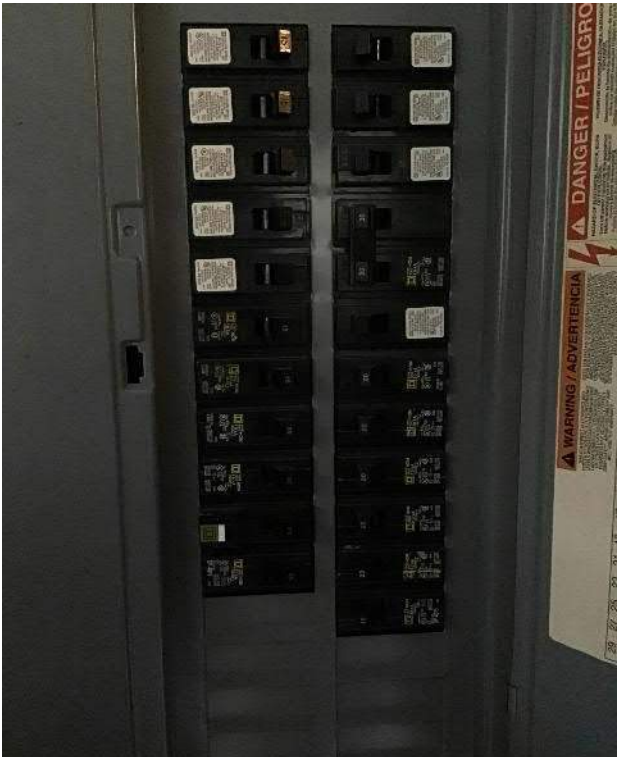
View of breaker box circuit breakers.
