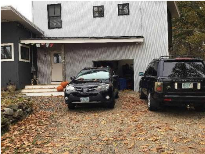
View of 74 Wentworth House Road and approximate location of the septic tank under the cars, facing South.
