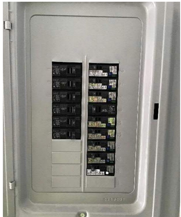
View of breaker box #2 (Siemens) circuit breakers.
