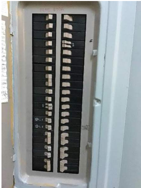
View of breaker box #3 circuit breakers.
