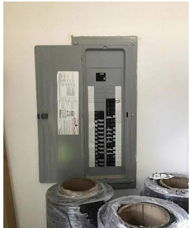
View of breaker box #2 (Siemens) located on the wall of the garage, facing Southeast.
