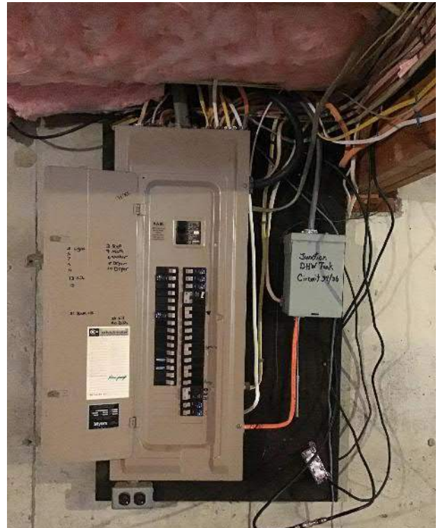
View of the breaker box and surrounding wall space facing Northeast.
