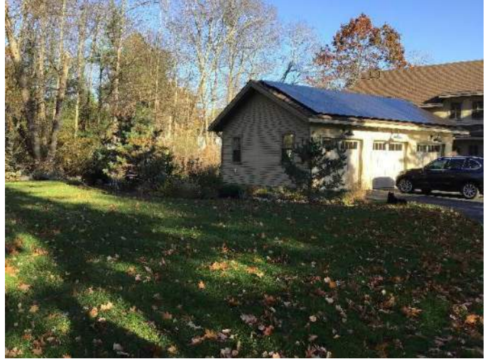
View of front yard and rain garden adjacent to the garage facing East.
