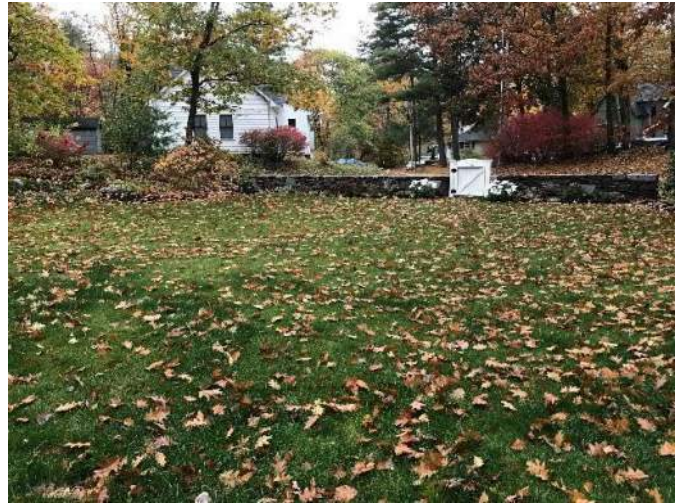
View of retaining wall crossing the proposed sewer service pathway facing West.
