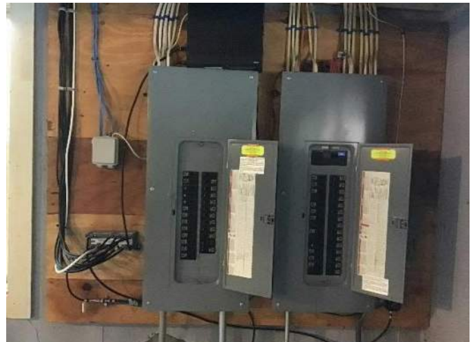
View of breaker boxes (#1 on left) and surrounding wall space located in the garage, facing Northeast.
