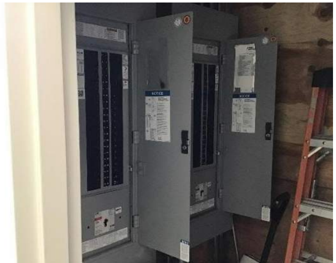
View of breaker box #1 on the left and #2 on the right, located in a closet on the West portion of the building closest to Sagamore Ave. facing Northwest.
