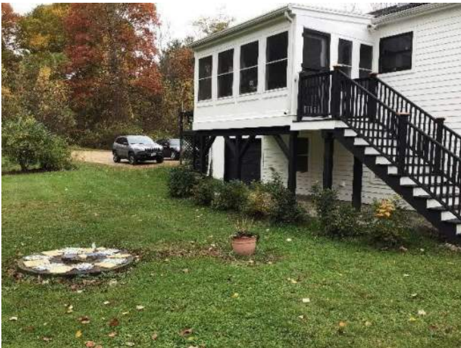
View of rear porch and wooden stairs with shrubs located beneath, facing West.
