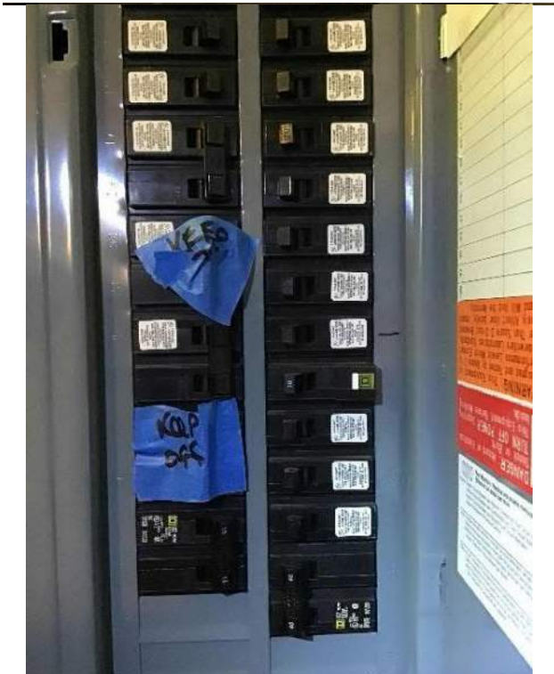
Continued view of breaker box #2 circuit breakers.
