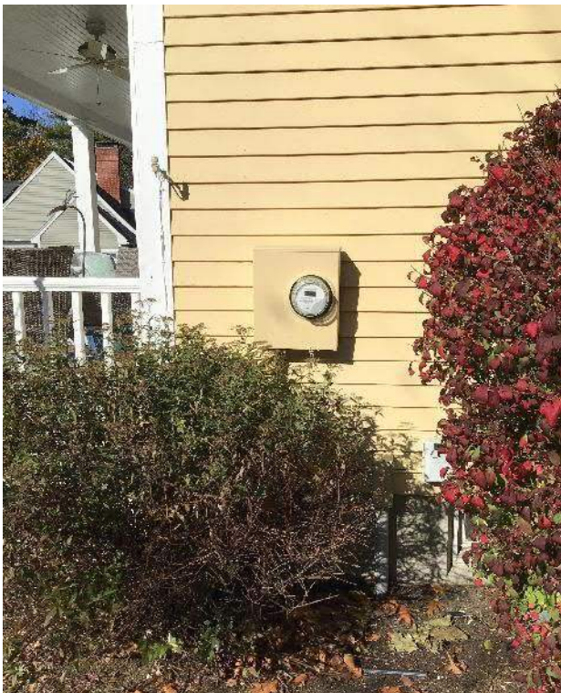
View of Southeast side of the house and breaker box location from the outside, facing Northwest.
