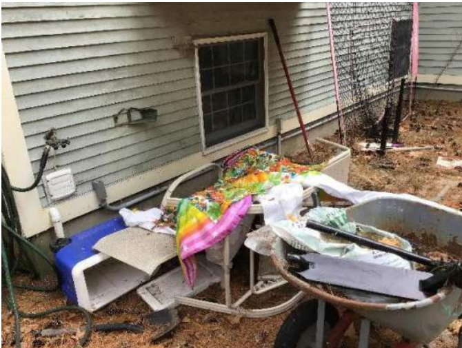
View of approximate location of buried sewer lateral, facing East.
