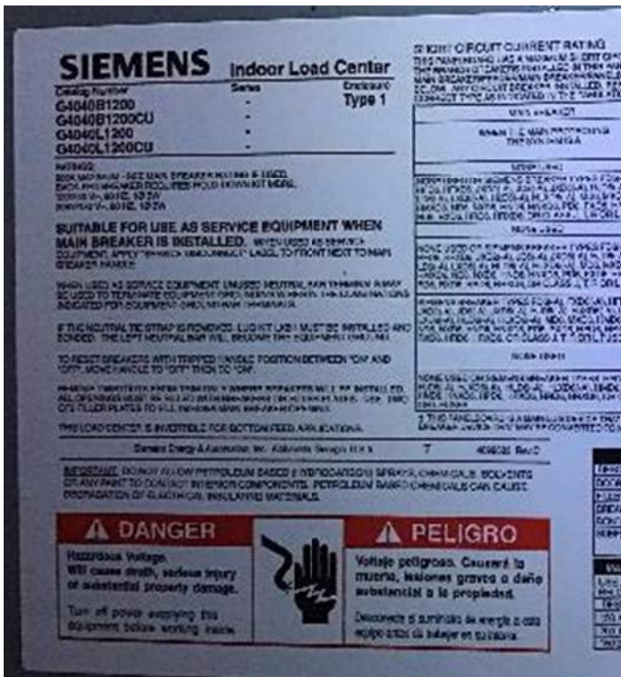
View of breaker box #1 model information and specifications.
