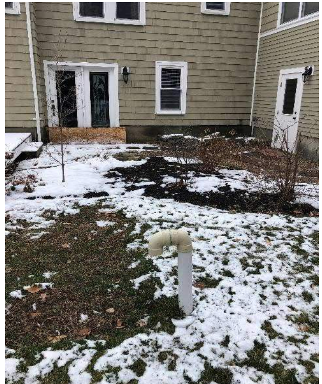
View of approximate location of the septic tank and pump station buried in the backyard, facing
