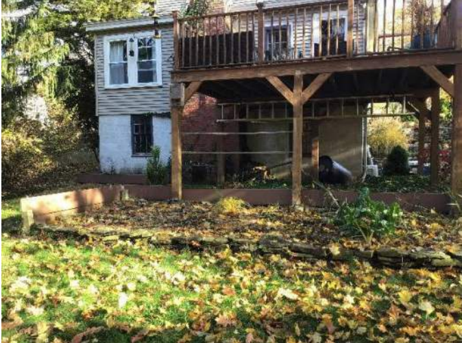
View of raised wooden porch and large planter box along the proposed sewer service pathway, facing Northeast.
