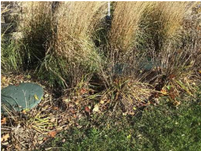
View of septic tank caps hidden within the shrubs on the West side of the building facing East.
