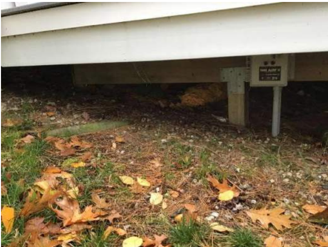
View underneath the wooden deck with sewer lateral and tank alarm system, facing Southwest.
