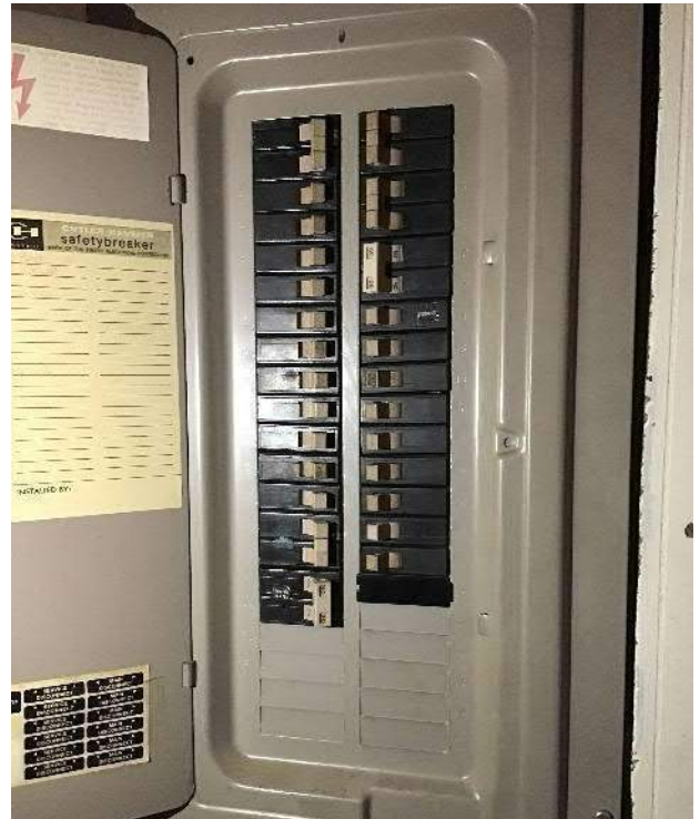
View of breaker box #1 circuit breakers.
