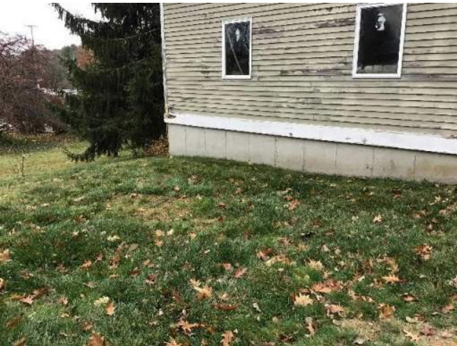
View of the approximate location of buried septic tank adjacent to garage building facing South.
