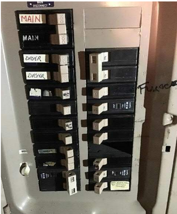
View of breaker box #1 circuit breakers with some schedule labels on the breaker switches.
