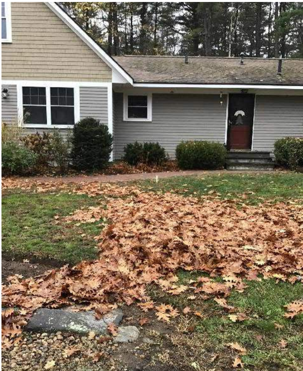
View of approximate water service location running underneath a brick walkway facing Southwest.
