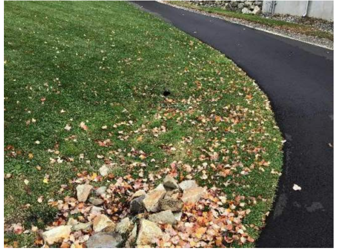
View of storm drainpipe along driveway and rocks for erosion control facing Northeast.
