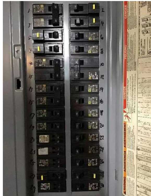
View of breaker box #1 circuit breakers.
