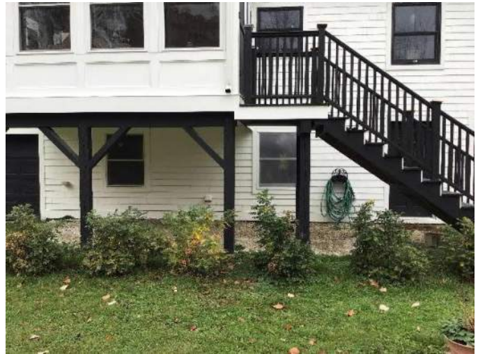
View of approximate location of the buried sewer lateral exiting the rear of the house facing Northwest.
