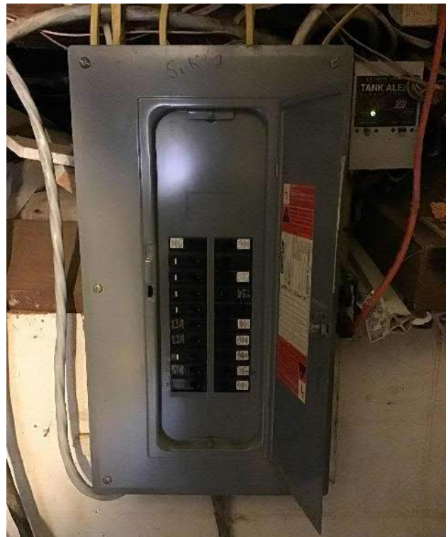
View of breaker box #1 in unfinished basement adjacent to PVC sewer lateral facing Northeast.
