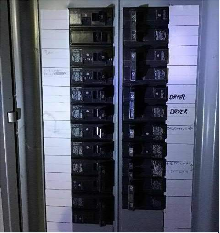
View of breaker box #1 circuit breakers and schedule adjacent to breaker switches.
