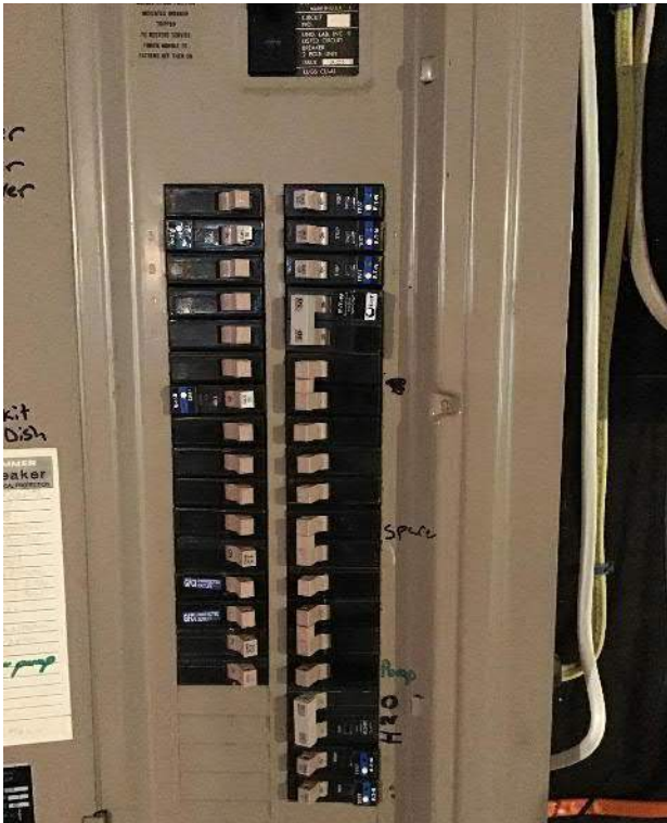
View breaker box circuit breakers.
