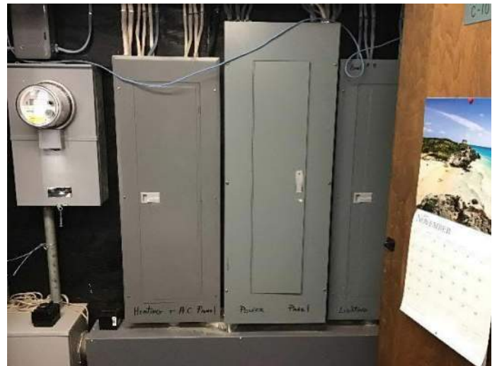
View of breaker box #4 and #5 on the right located in a closet near the Southwest exit from the building facing South.
