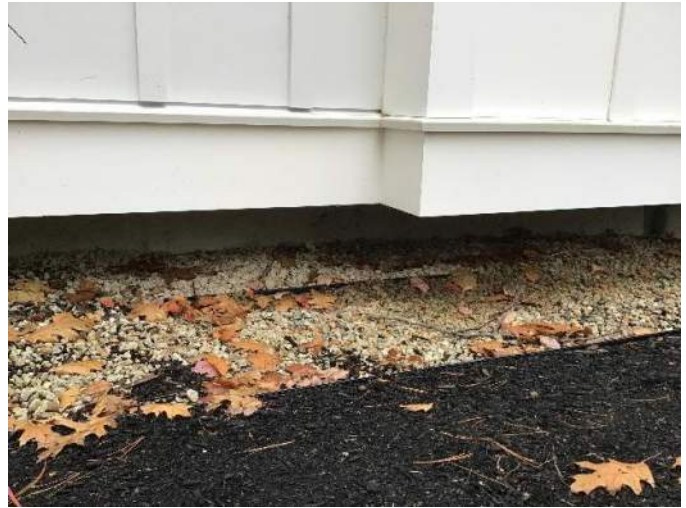
View of approximate location of the buried sewer lateral exiting the foundation, facing Southeast.
