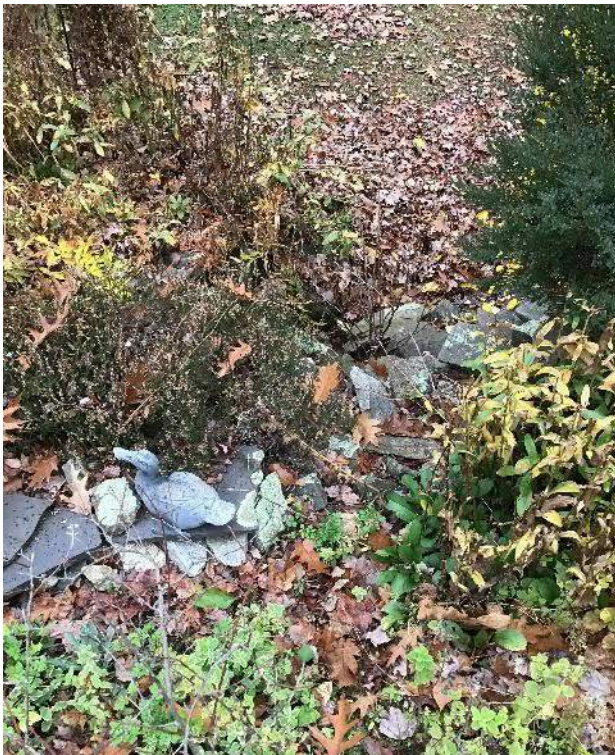
View of the top of the culvert facing Northwest.
