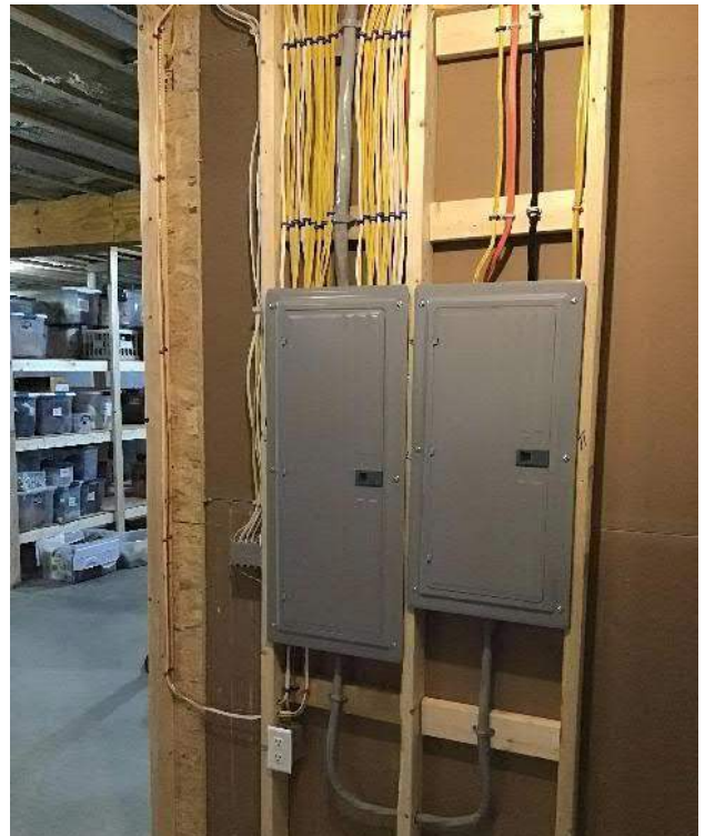
View of two breaker boxes (#1 is left) and surrounding wall space facing West.
