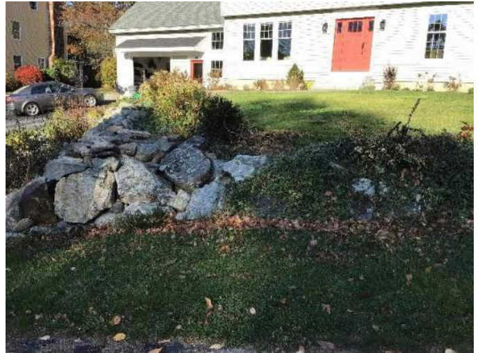
View of the front yard and large retaining wall sloping towards the road, facing North.
