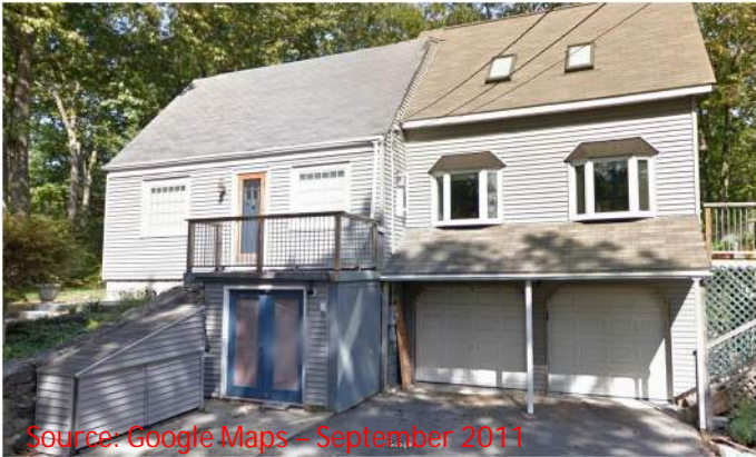
View of 171 Walker Bungalow Road from the road facing Northeast.
