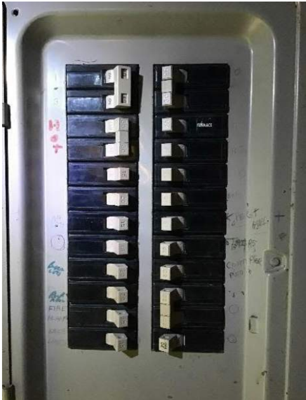
View of breaker box #2 circuit breakers located on the wall in the first-floor main lobby.
