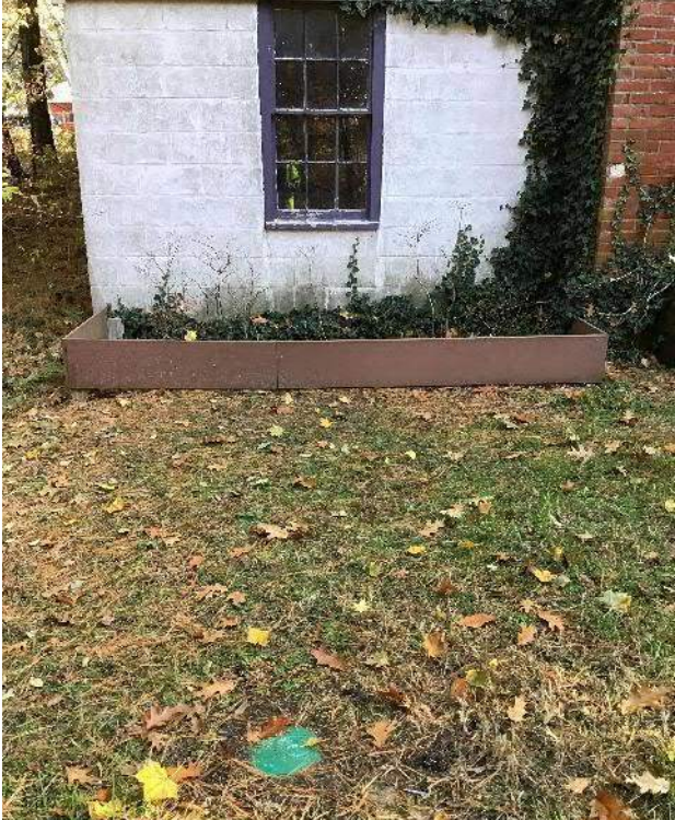
View approximate sewer lateral location with septic tank cap in the foreground, facing Northeast.
