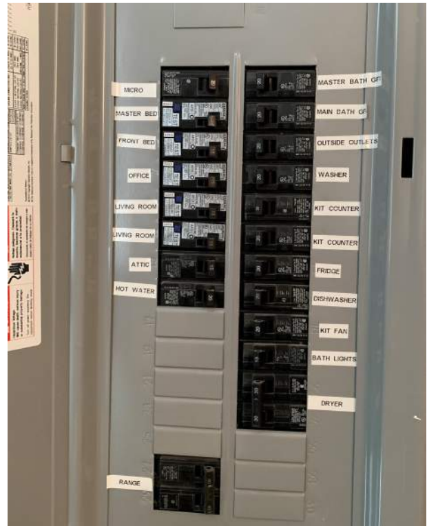
View of breaker box #1 circuit breakers and schedule adjacent to the breaker switches.
