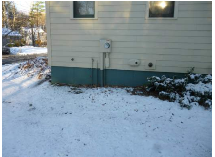
View of the electricity meter on the Southeast side of the house, facing Northwest.
