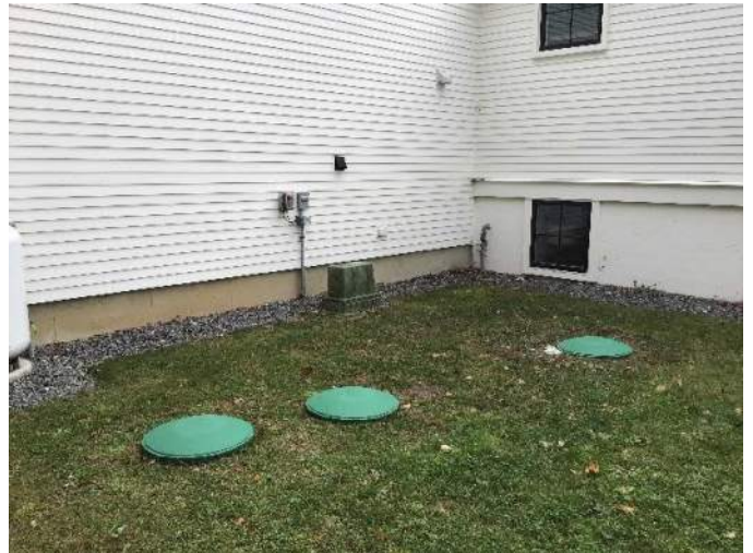
View of septic tank and caps behind the West side of the house facing Southeast.
