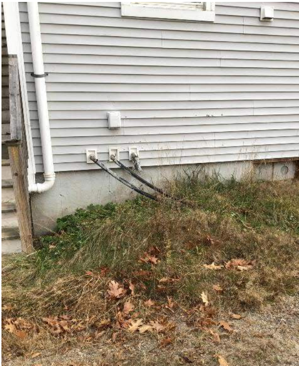
View of approximate existing sewer lateral location facing South.
