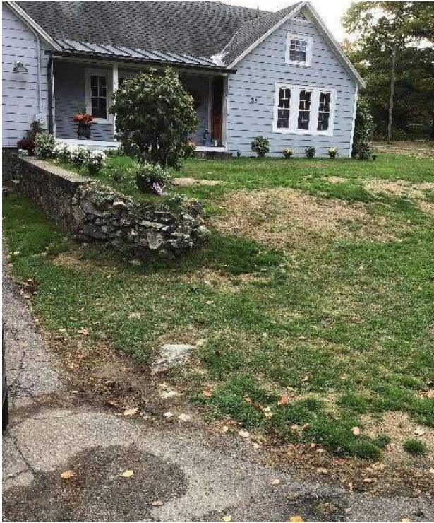
View of 33 Cliff Road from the road facing South.
