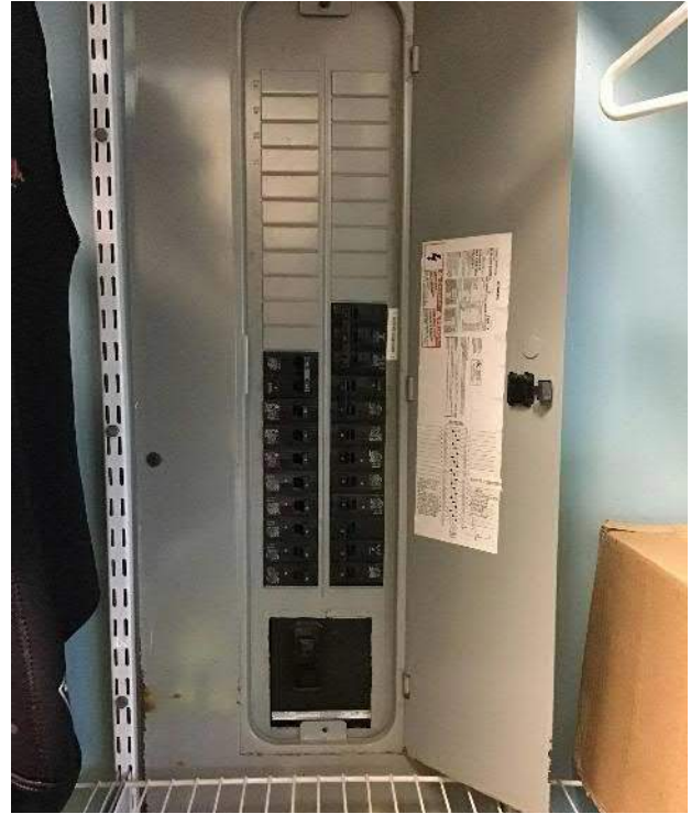
View of breaker box #1 and surrounded wall space located in a closet on the first floor facing Northwest.
