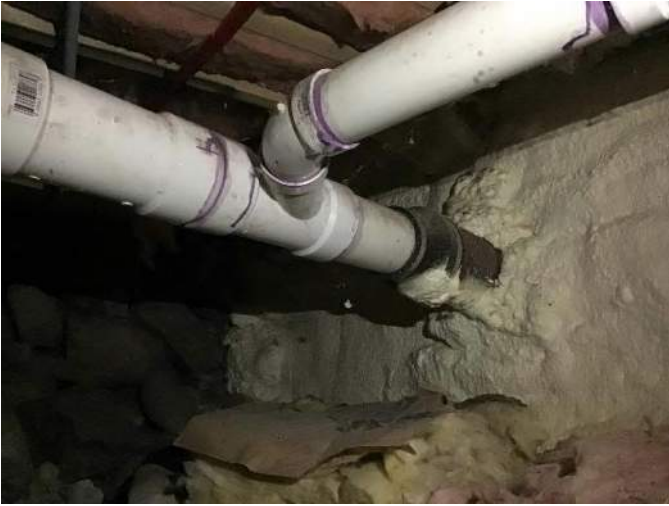
View of exposed cast iron lateral exiting the foundation to the backyard, facing Southeast.
