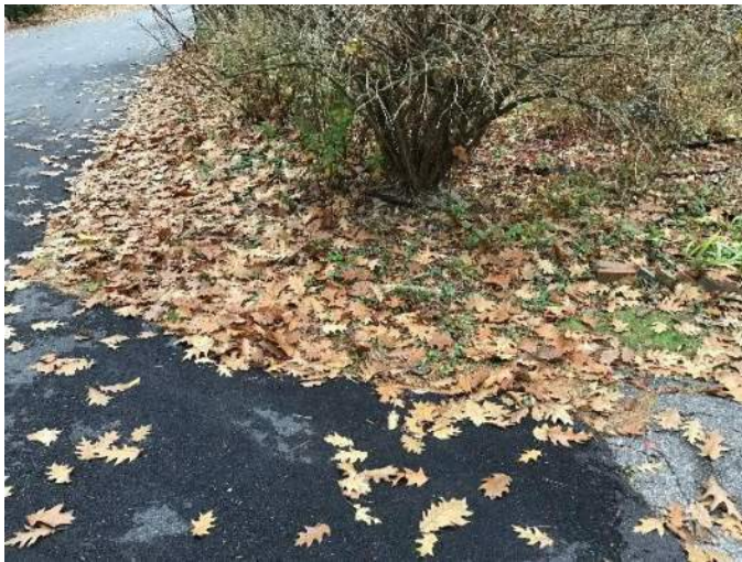
View of asphalt apron and shrub adjacent to the entrance to the driveway facing Southeast.
