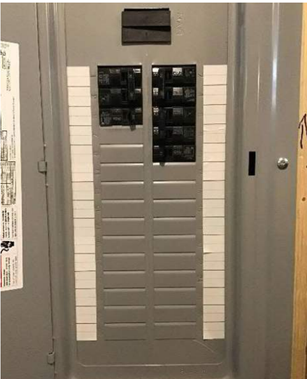
View of breaker box #2 circuit breakers.
