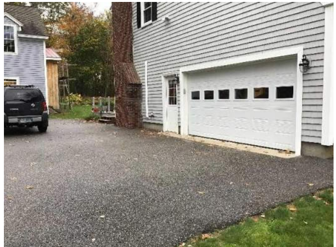
View of asphalt driveway and concrete apron for the garage, facing Northwest.
