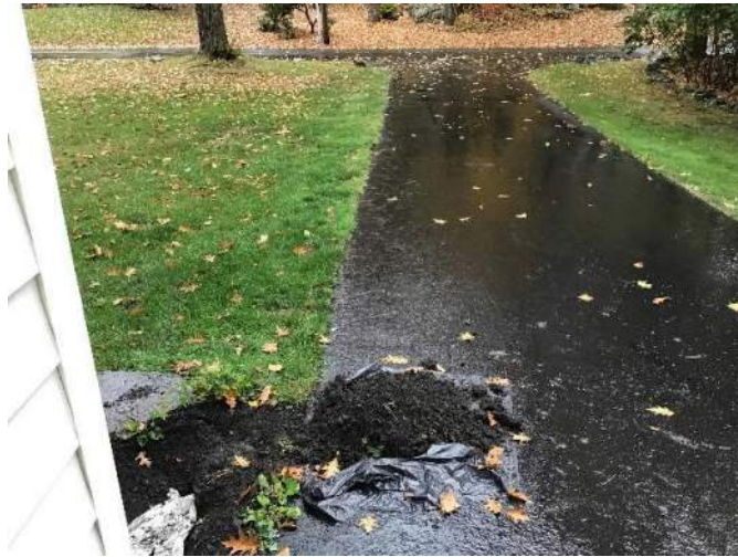
View of the second septic tank with landscaping removed, located on the Northeast side of the house adjacent to the garage and driveway facing Northeast.
