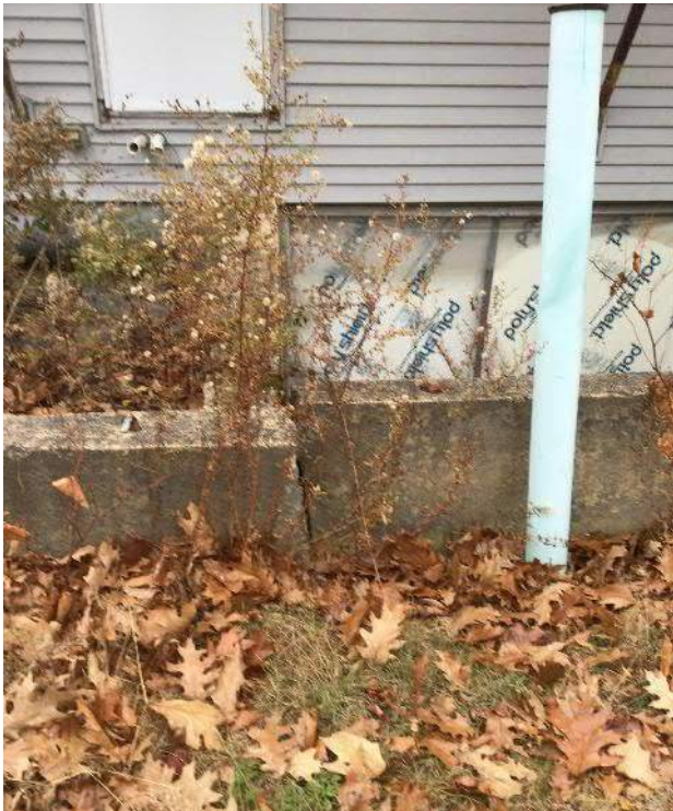
View of crack in the concrete retaining wall due to overturning facing Southwest.
