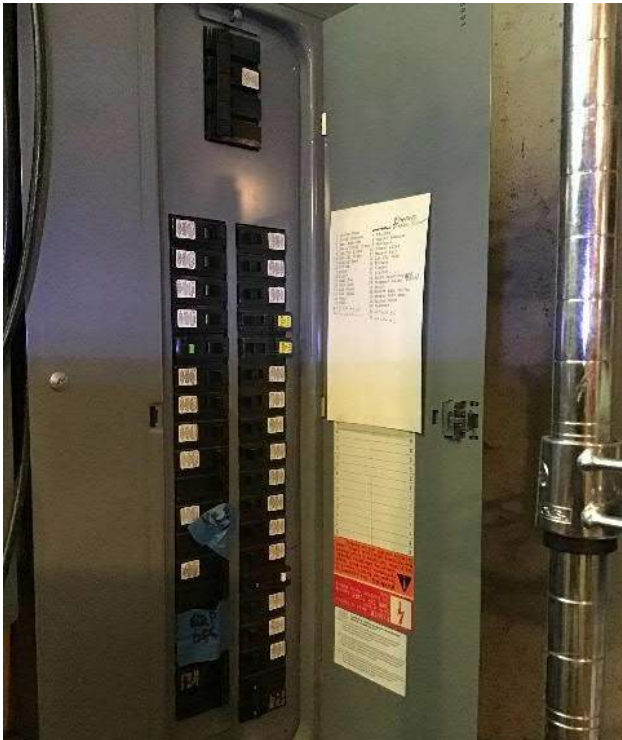
View of breaker box #2 front panel open.
