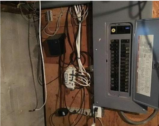
View of breaker box #1 and surrounding wall space located on the South foundation wall in the basement, facing South.
