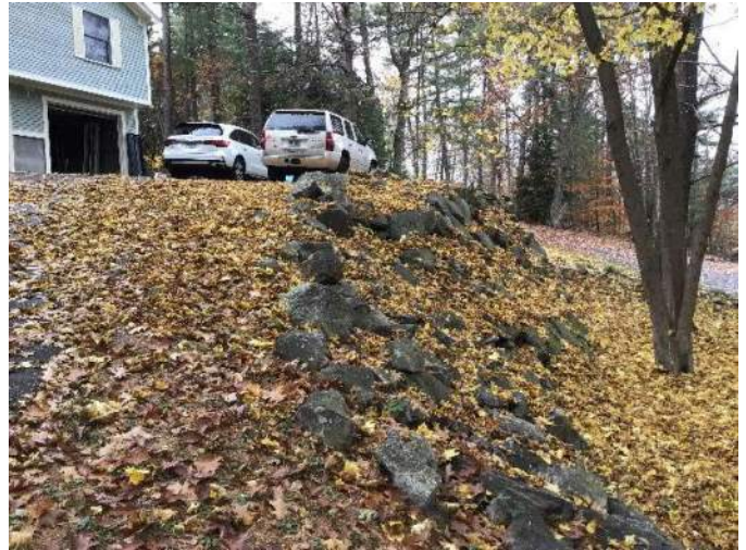
View of retaining wall and asphalt driveway facing Northwest.
