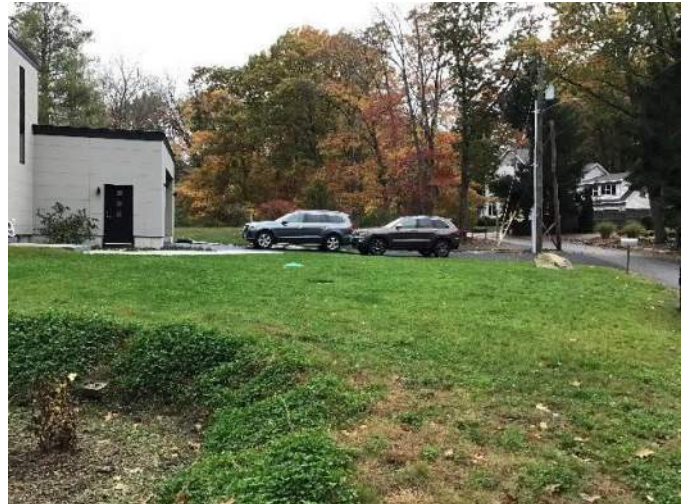
View of the front yard and holding tank cap in the middle facing West.
