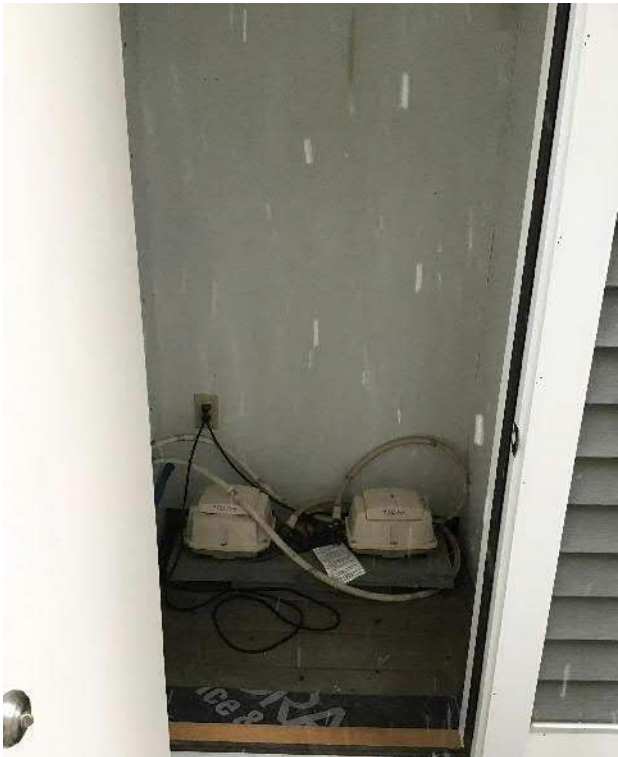
View within the "Septic Controls" room facing Southeast.
