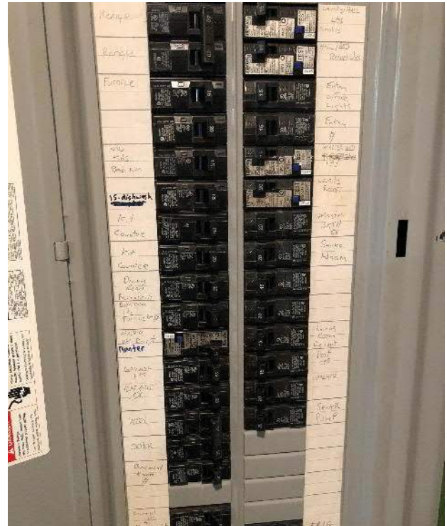
View of Siemens breaker box circuit breakers and schedule adjacent to breaker switches.
