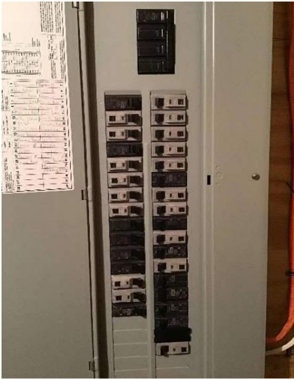
View of breaker box circuit breakers.
