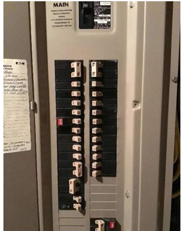
View of the breaker box circuit breakers.
