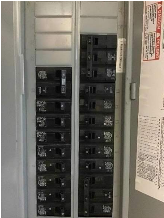
View of breaker box #1 circuit breakers.
