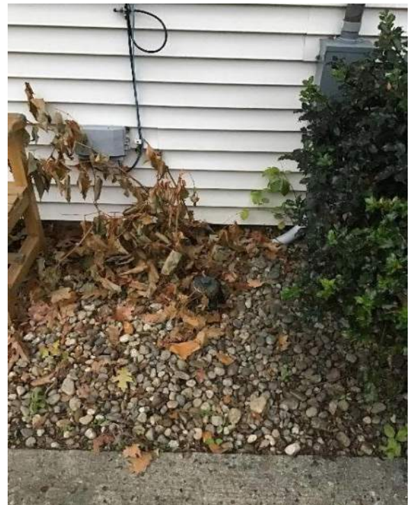
View of sewer lateral exiting the concrete foundation and cleanout between a bench and bush facing North.
