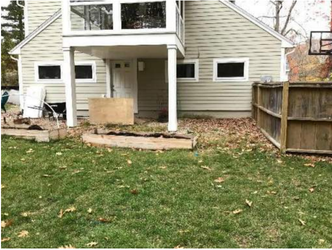
View of buried septic tank, sewer lateral location and planter boxes set up on top, facing Northwest.
