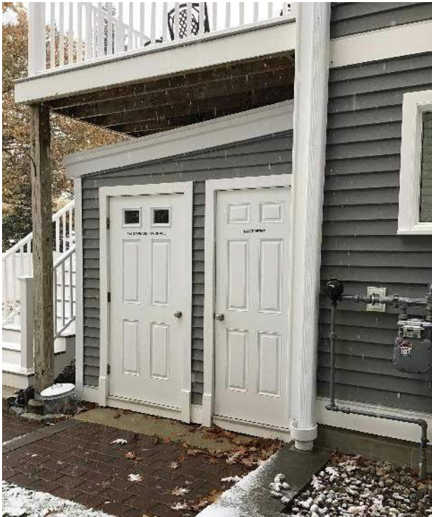
View of raised porch, brick path, and doors to access utilities facing East.
