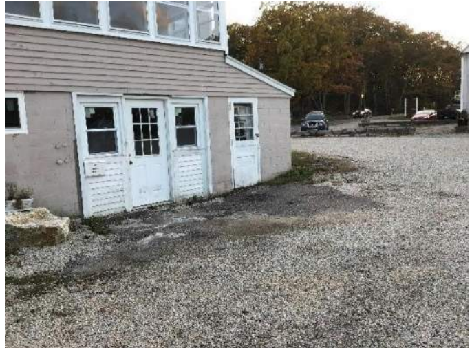
View of the rear side of the house standing in the gravel parking lot facing Southwest.
