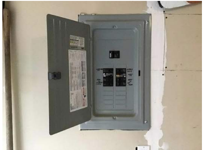
View of breaker box #2 (Siemens) and surrounding wall space located on the West wall of the garage facing West.
