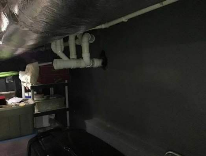
View of the sewer lateral located in the basement exiting into the Southwest concrete foundation facing South.
