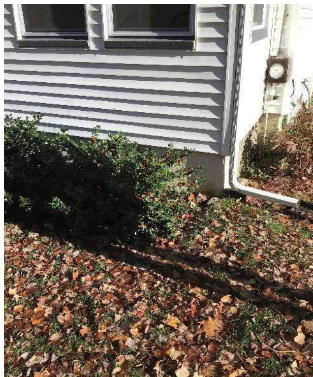
View of small shrubs along the front of the house facing Northeast.
