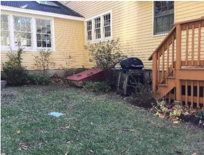
View of approximate location of the sewer lateral just beyond the bulkhead door facing Southeast.
