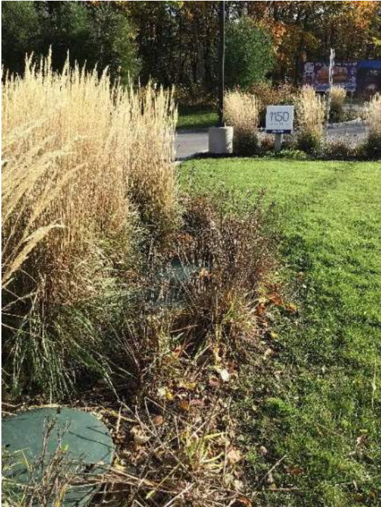
View of holding tank caps within the shrubs on the West side of the building facing South.
