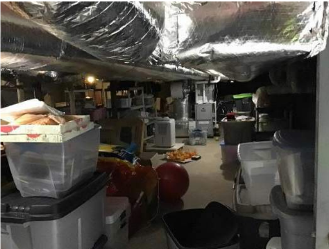
View of the basement from the bulkhead stairs looking towards the breaker box in the East corner facing Southeast.
