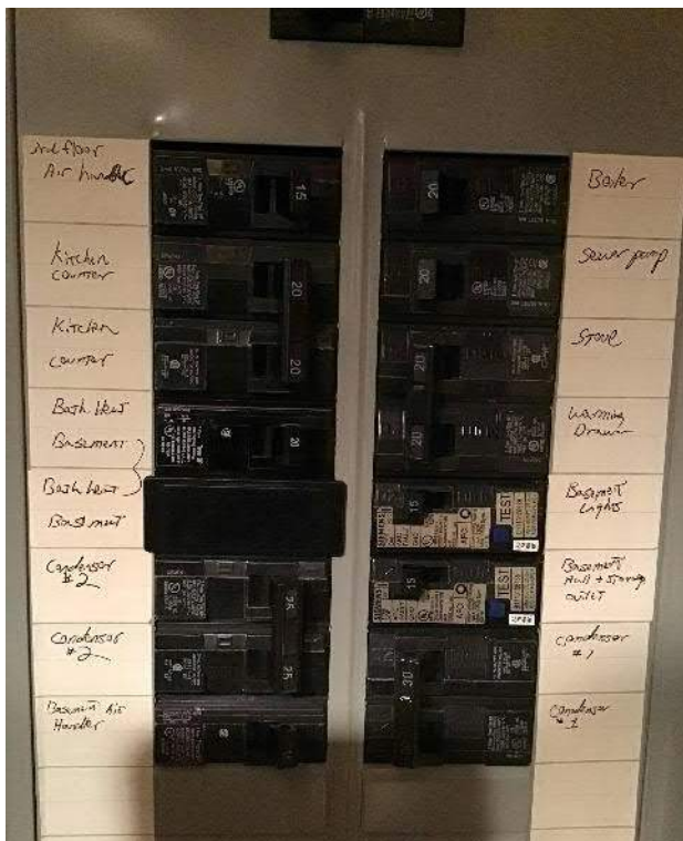
View of breaker box #2 circuit breakers and schedule adjacent to the breakers.
