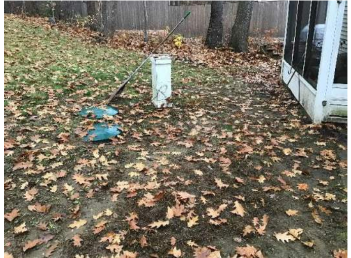
View of approximate location of the buried sewer lateral and covers for the septic tank and pump station facing East.
