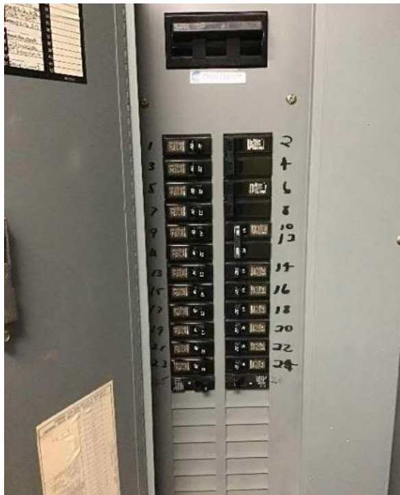
View of breaker box #4 (Challenger) circuit breakers located near the Southwest exit from the building facing South
