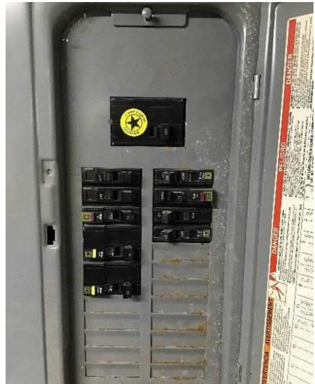
View of breaker box #1 circuit breakers and available slots.
