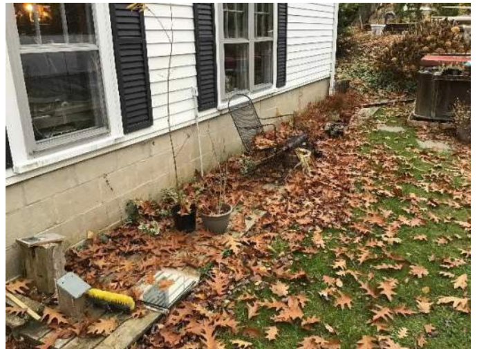
View of approximate location of buried sewer lateral facing Northwest.
