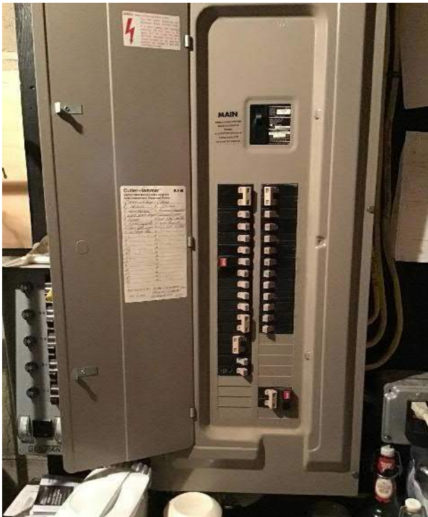
View of the breaker box located in a closet on the ground floor, facing Northwest.
