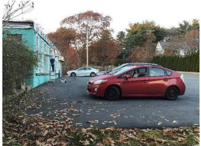
View of proposed sewer service path along the front of the building facing Northwest.
