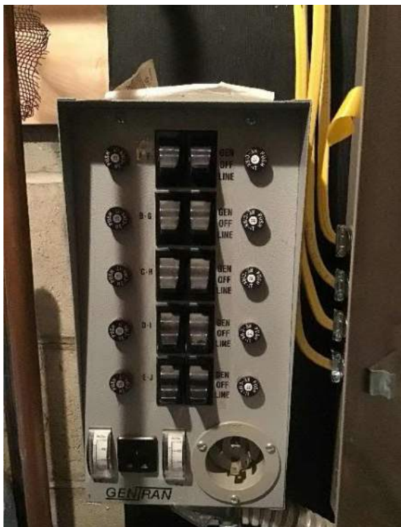
View of manual transfer switch front panel to the left of the breaker box.
