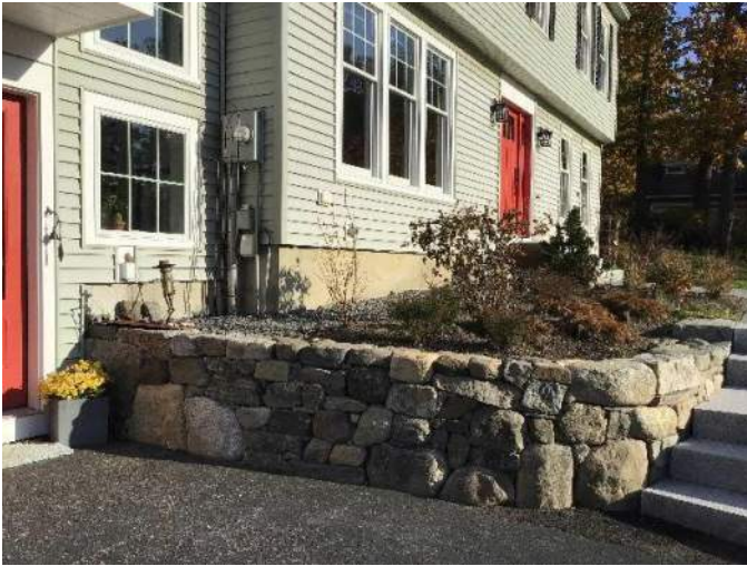
View of 290 Walker Bungalow Road from the driveway facing East.
