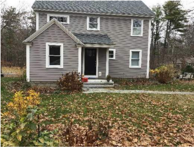
View of 71 Cliff Road from the road facing Northeast.
