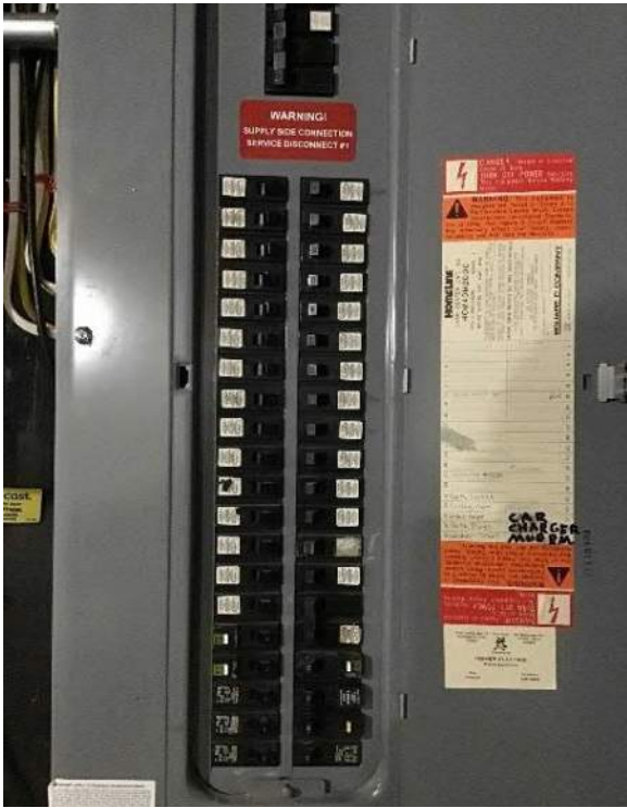
View of breaker box circuit breakers.
