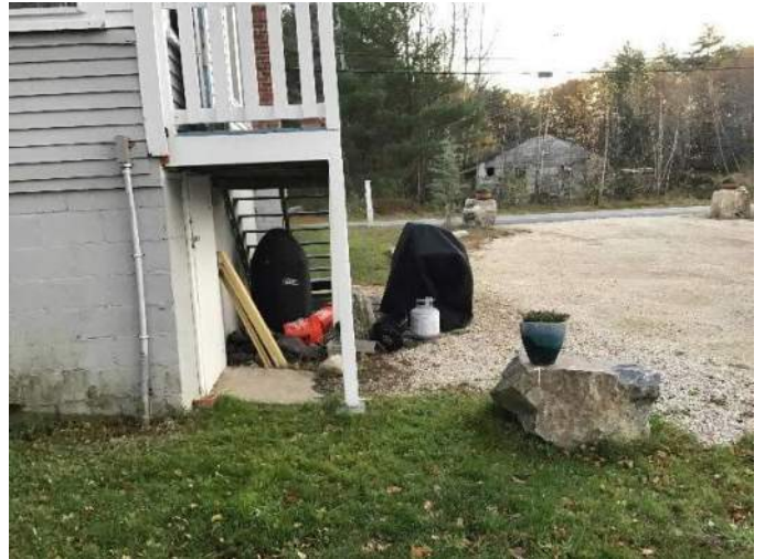
View of proposed sewer service path towards the road facing South.
