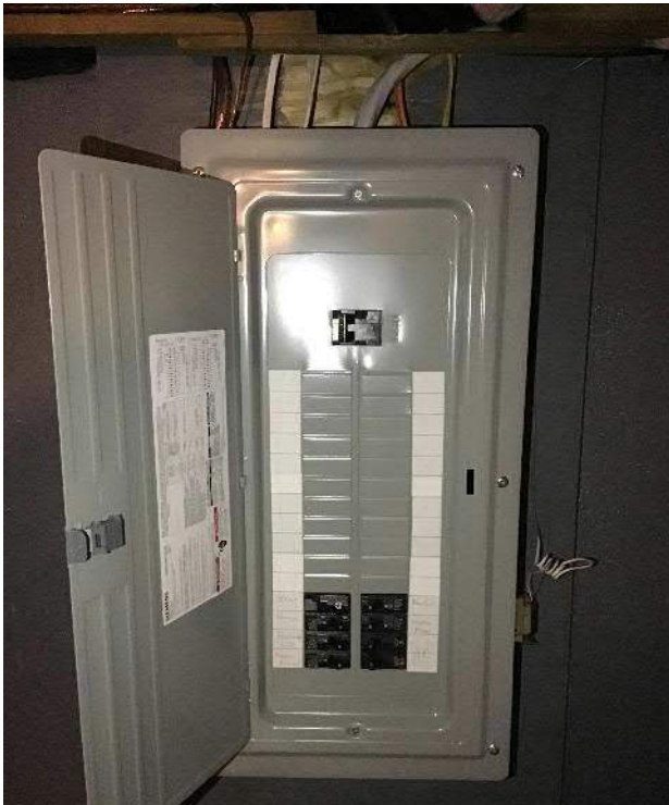
View of breaker box #1 located in the East corner of the basement, facing Southeast.
