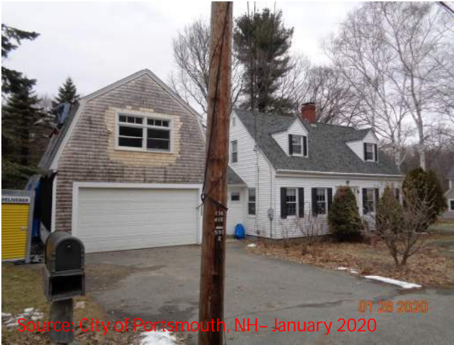
View of 44 Cliff Road from the road, facing North.
