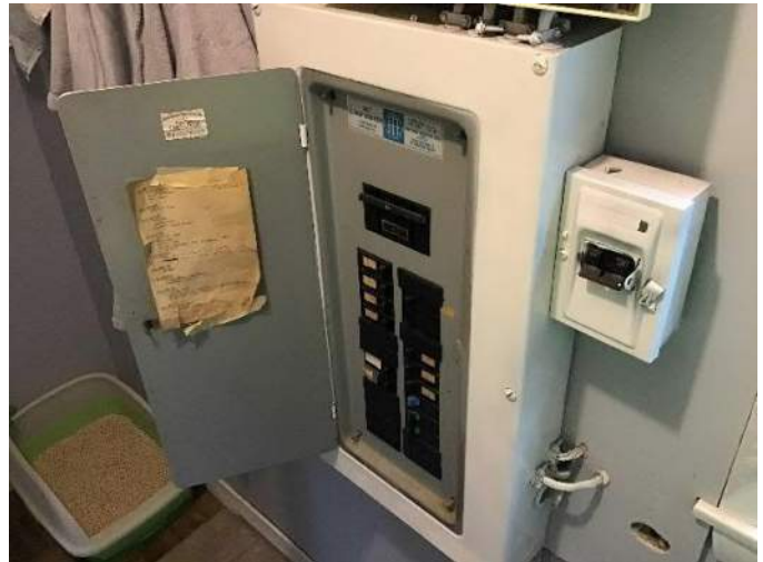
View of the breaker box located in the bathroom facing East.
