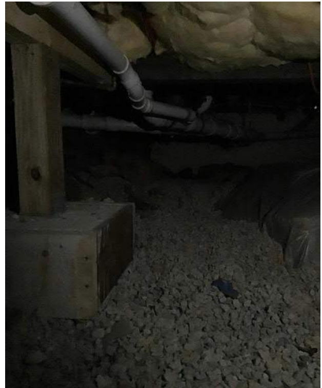
View of PVC plumbing located in the crawlspace underneath the house facing South.
