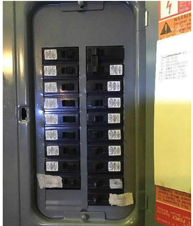
View of breaker box #1 circuit breakers.
