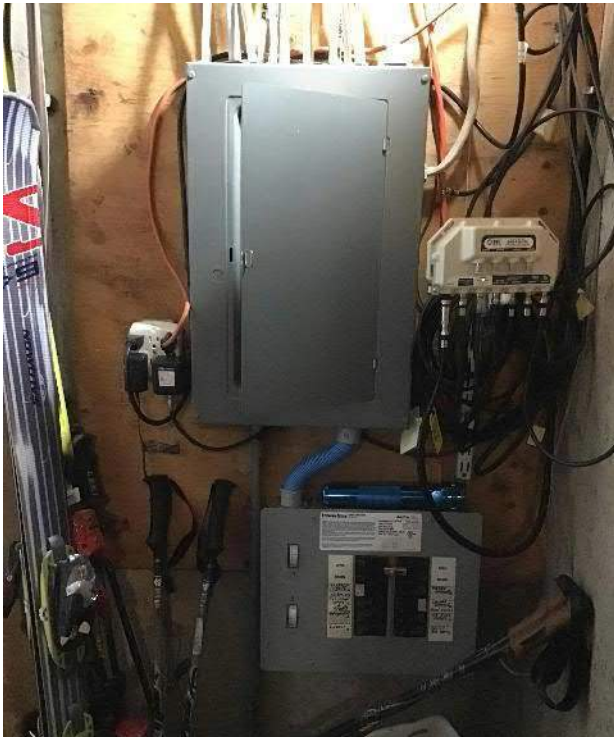
View of the surrounding wall space around the breaker box and transfer switch facing Northwest
