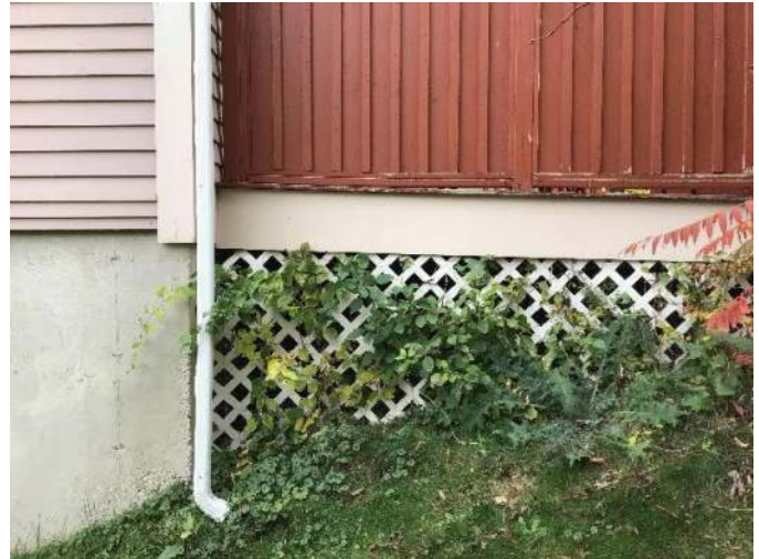
View of sewer lateral located under the wooden porch and behind the lattice, facing Southwest.
