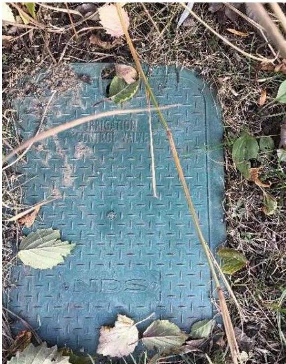
View of buried irrigation system on the Northwest corner of the building close to the intersection facing East.
