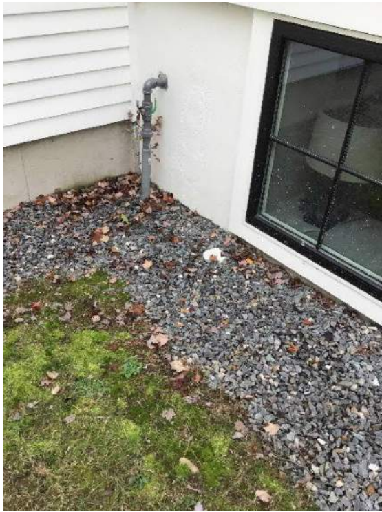
View of approximate location of buried sewer lateral facing Southeast.
