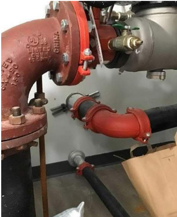
View of fire suppression system in a closet on the West section of the building facing Northwest.
