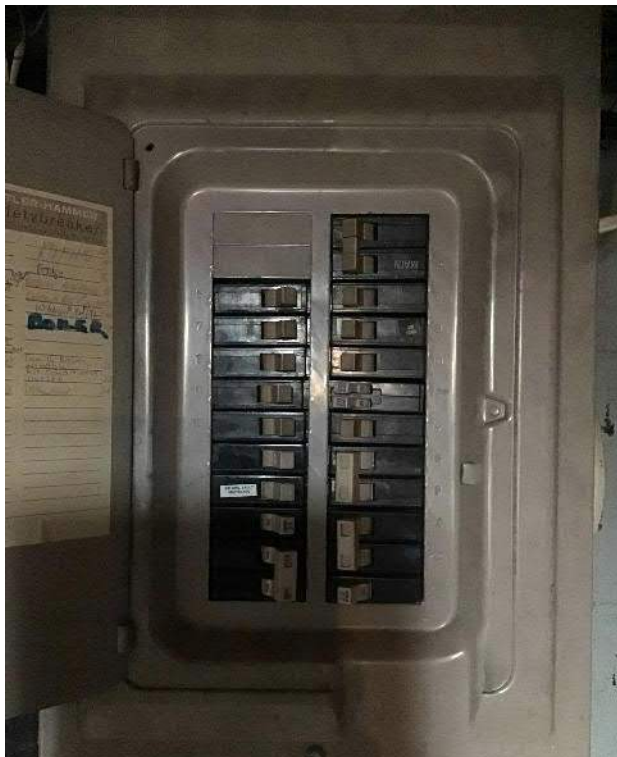
View of breaker box circuit breakers.
