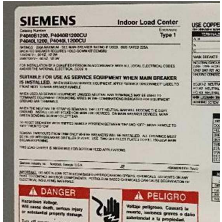
View of breaker box #1 model information and specifications.
