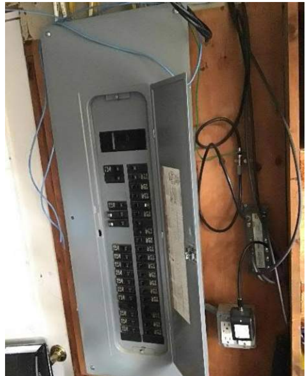
View of the breaker box and surrounding wall space located next to the door in the garage facing Northeast.
