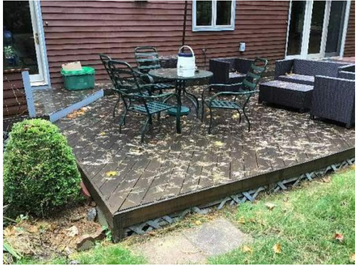
View of wooden deck covering the location of where the buried sewer lateral exits the foundation facing East.
