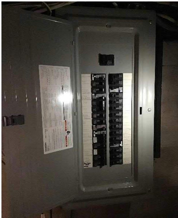
View of the breaker box with the front panel cover open, facing Southeast.
