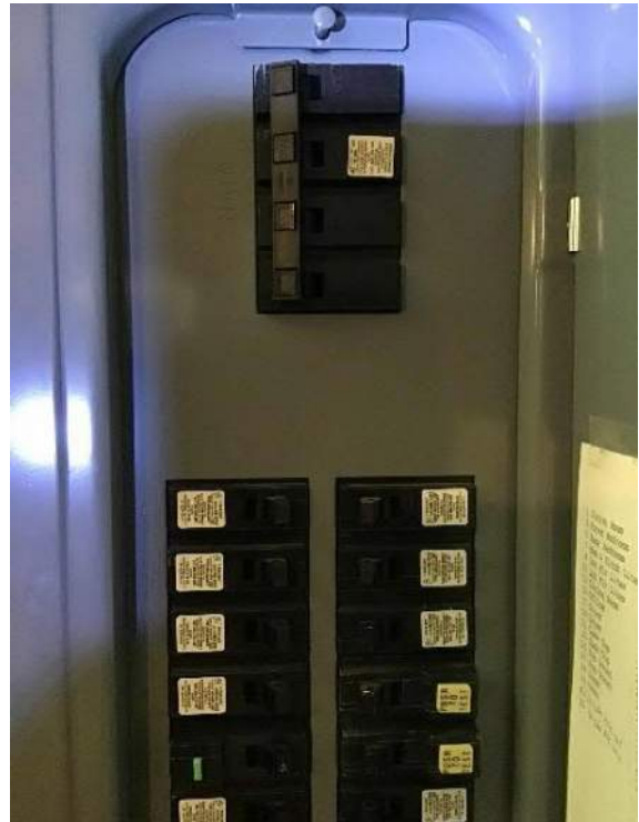
View of breaker box #2 circuit breakers.
