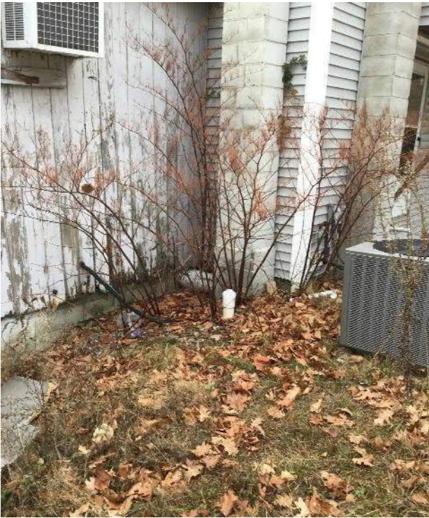
View of PVC cleanout behind the building near shrubs and an AC unit facing West.
