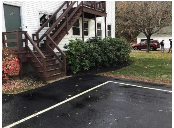
View of shrubs and mulch against the North wall of the building on top of sewer lateral facing Southwest.
