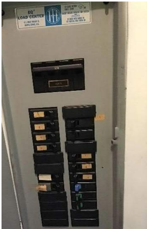
View of breaker box circuit breakers and model information at the top.
