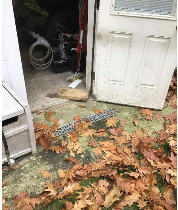
View of small channel drain outside of the rear basement door facing West.
