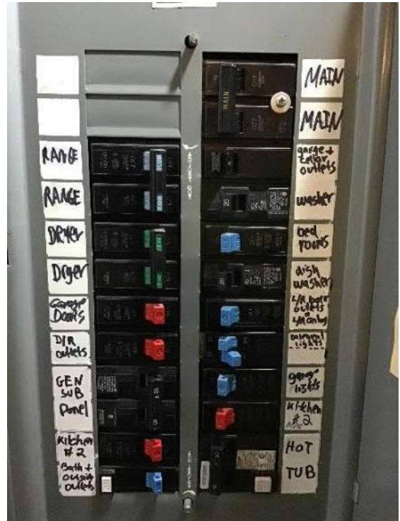
View of circuit breakers and schedule adjacent to breaker switches.
