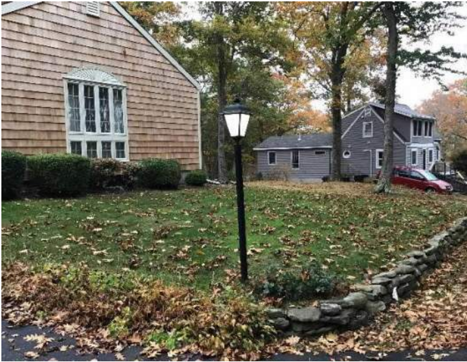
View of 159 Walker Bungalow Road and buried septic tank off the Southwest corner of the house, adjacent to the asphalt driveway facing East.
