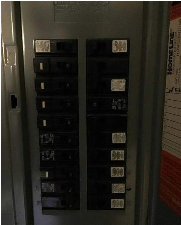
View of breaker box #1 circuit breakers.
