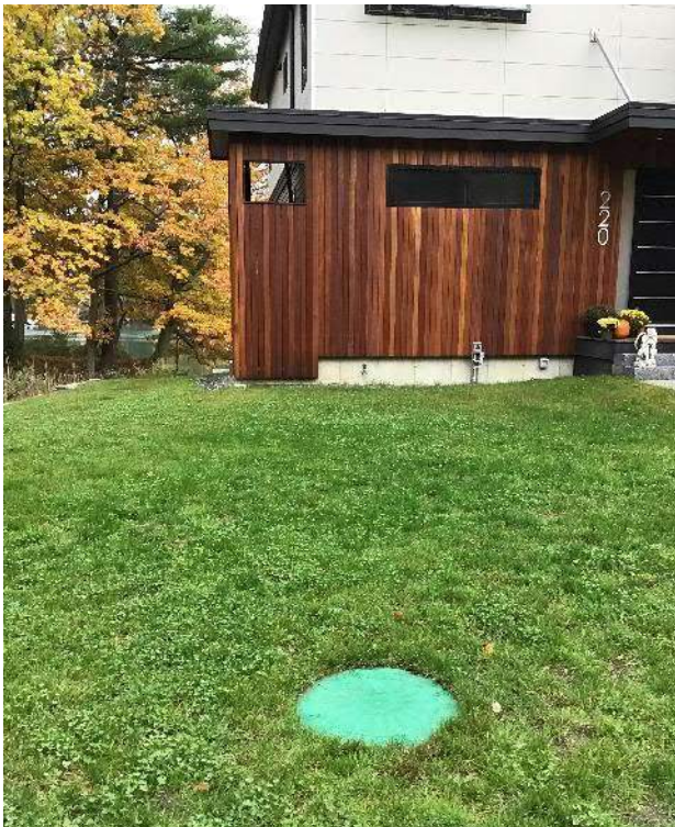
View of holding tank cap and location of buried sewer lateral facing South.
