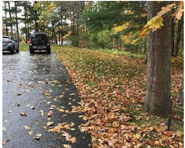
View of lawn and tree adjacent the driveway and location of proposed sewer service, facing Northeast.
