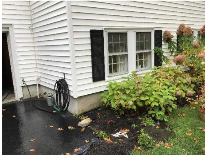
View of the second septic tank with landscaping removed to clean out the tank, located on the Northeast side of the house facing Walker Bungalow Rd looking West.
