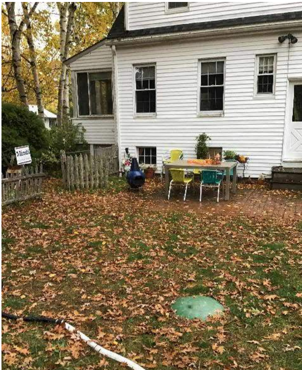
View of septic tank cap and approximate location of sewer lateral under wooden steps, facing Southeast.
