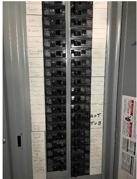
View of breaker box #1 circuit breakers and schedule, located in the garage, facing Southwest.
