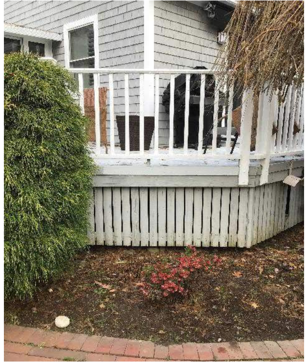
View of raised wooden deck and approximate location of the sewer lateral and septic tank underneath facing North.
