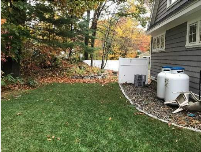
View of the Northwest yard and stone landscaping up against the house facing Northeast.
