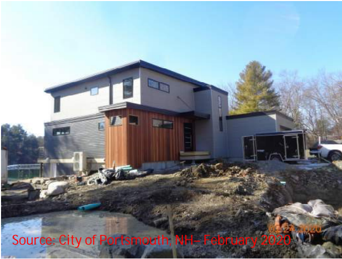
View of 220 Walker Bungalow Road facing Southwest.
