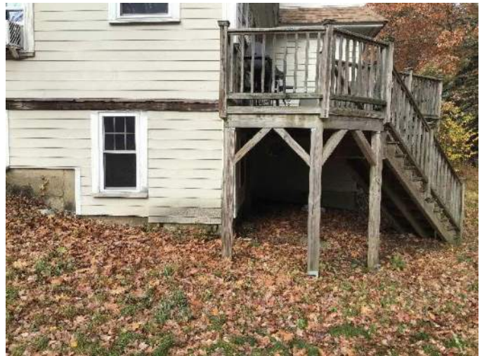
View of approximate buried sewer lateral location below the raised wooden porch, facing Northwest.
