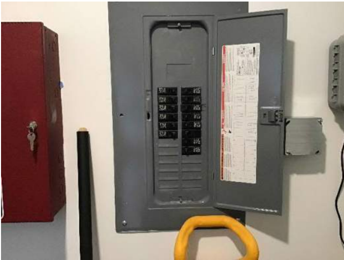
View of the breaker box and surrounding wall space located in a room on the South corner facing Northwest.
