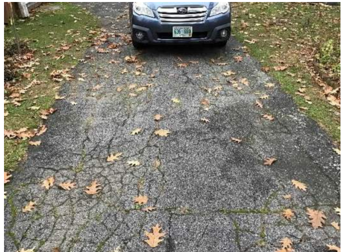
View of approximate location of drainage pipe running underneath the asphalt driveway facing Southwest.
