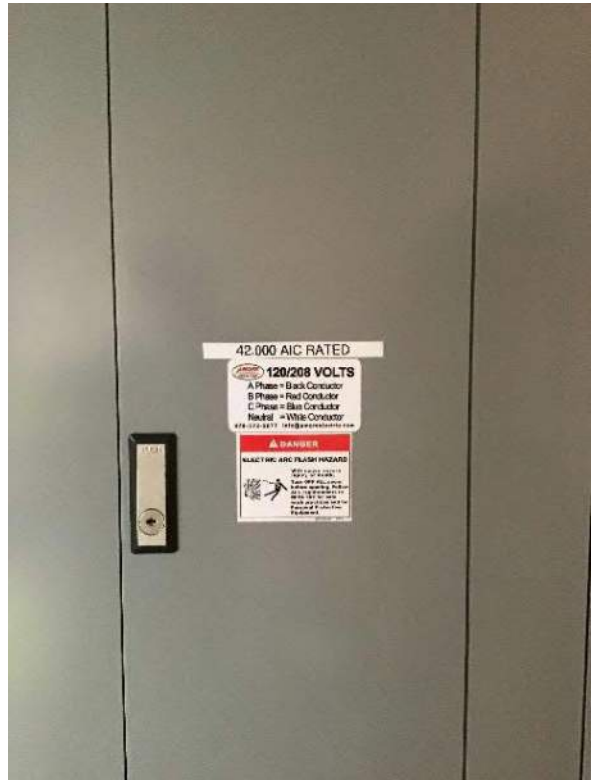
View of breaker box #2 exterior labels when closed.
