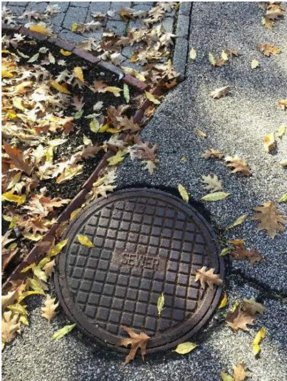
View of steel manhole cover for septic tank access facing South.
