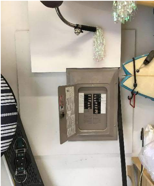
View of breaker box #2 and surrounding wall space located on the East interior garage wall, facing East.
