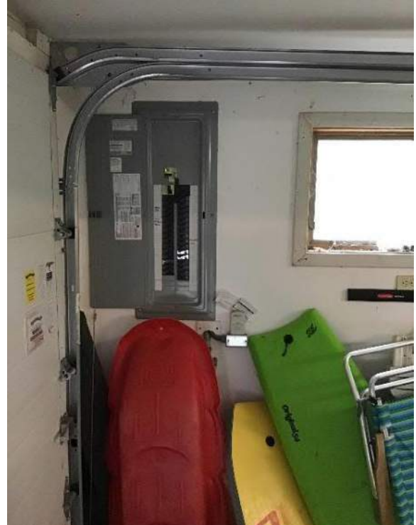
View of 200A breaker panel #1 wall space located on the Southeast exterior wall of the garage facing Southeast
