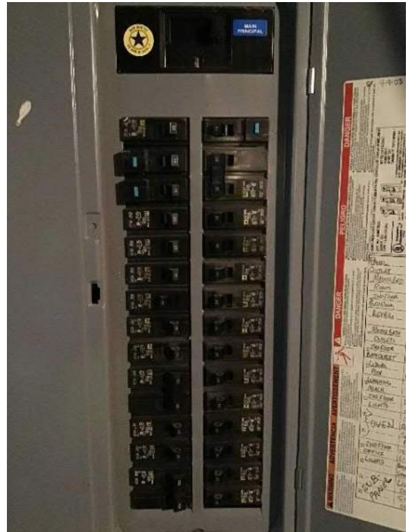
View of breaker box #1 circuit breakers.
