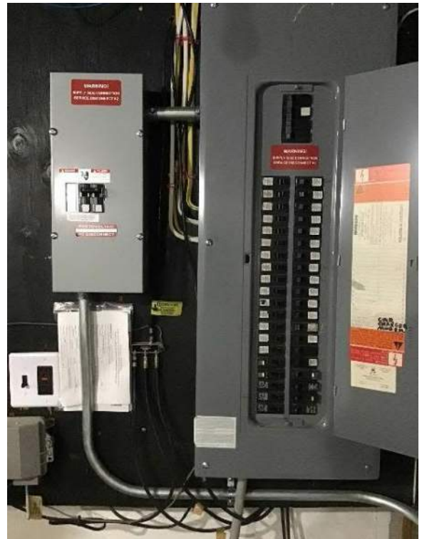
View of breaker box and AC photovoltaic disconnect facing Northeast.
