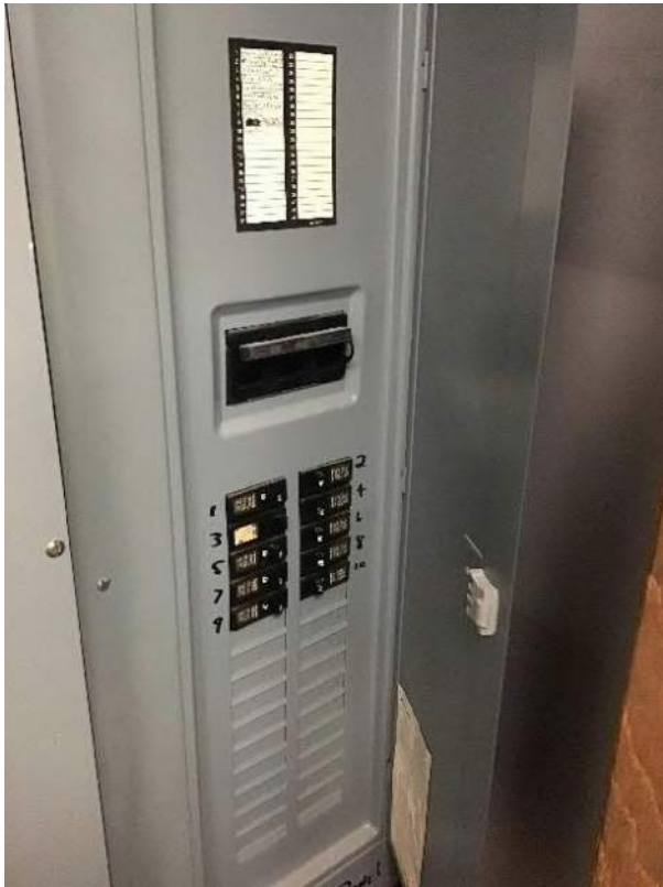
View of 200A breaker box #5 circuit breakers and schedule located to the right of box #4.
