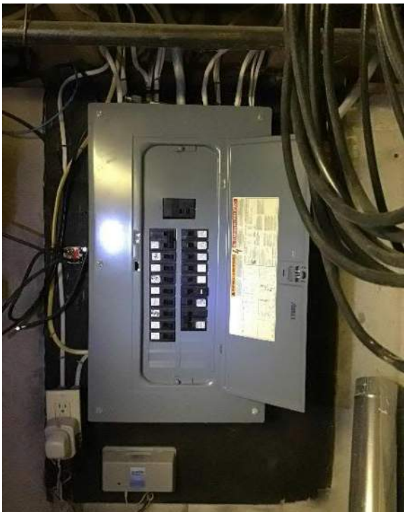
View of breaker box #2 and wall space in closet attached to the finished basement, facing North.
