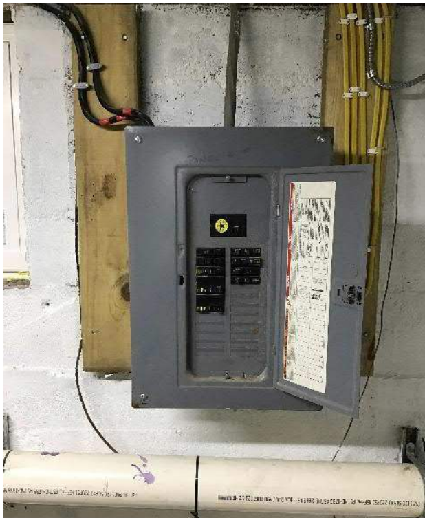
View of 100A breaker box #1 and surrounding wall space facing East.
