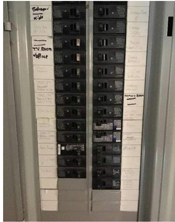
Continued view of 200A breaker box #1 circuit breakers and schedule adjacent to the breakers.
