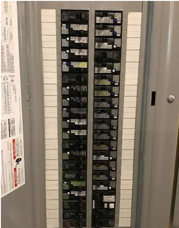
View of breaker box #1 circuit breakers.
