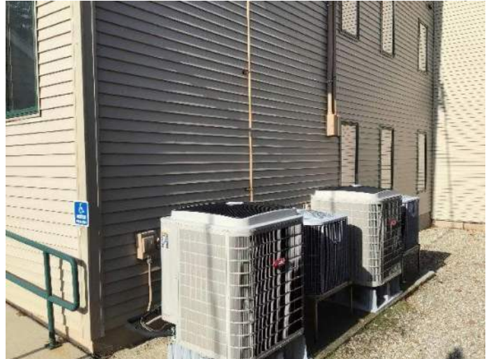
View of the Southwest exit and exterior location of breaker box #4 and #5 facing Northwest
