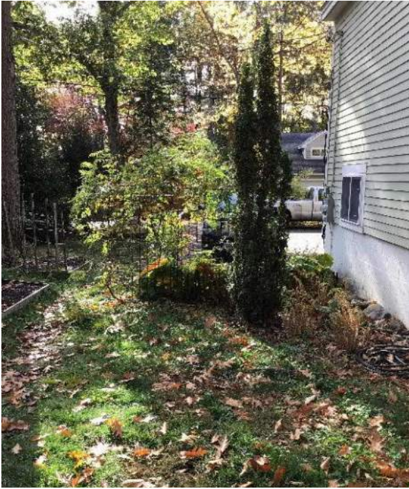
View of buried septic tank and lateral at the bottom of the frame standing adjacent to exterior garage wall facing Southwest.
