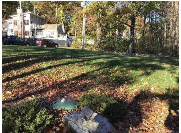
View of proposed sewer service pathway through the front yard leading towards the road, facing Northeast.
