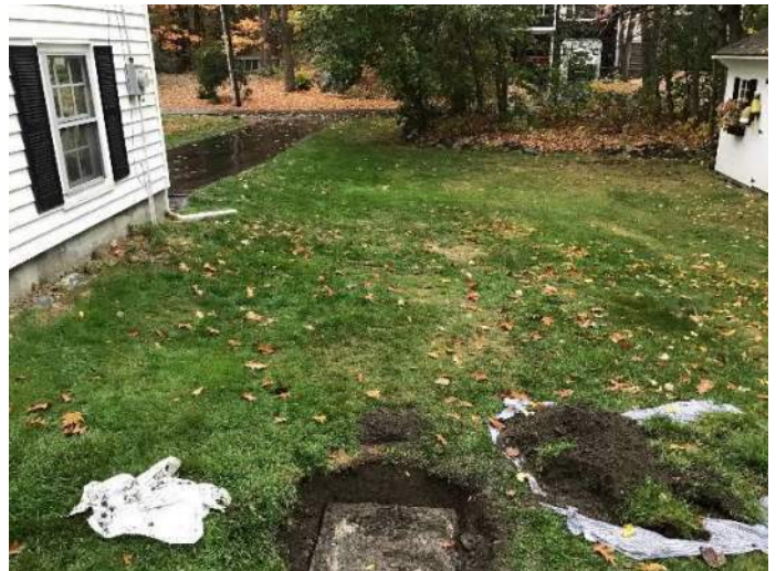
View of the first septic tank with turf removed to clean out the tank, located on the Southeast side of the house facing Northeast.
