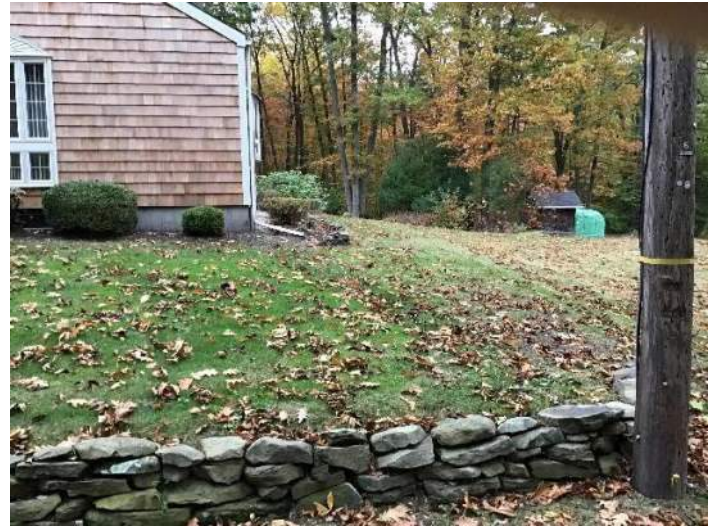
View of South corner of the house and with shrubs along the front and a retaining wall is in the forefront of the photo, facing Northeast.
