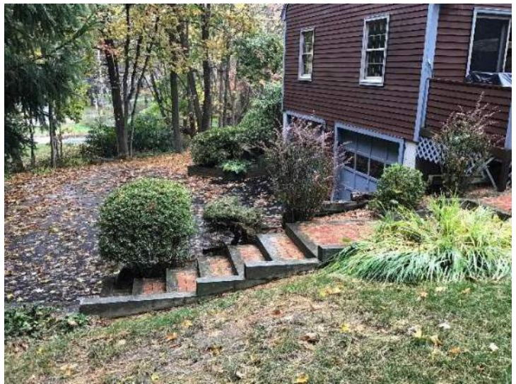
View of brick stairs and landscaping planted along the wooden retaining wall facing Northeast.
