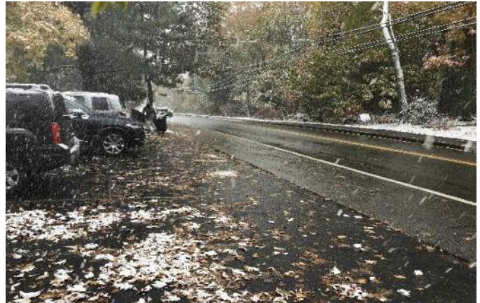
View of asphalt driveway sloping towards Sagamore Avenue facing Southeast.
