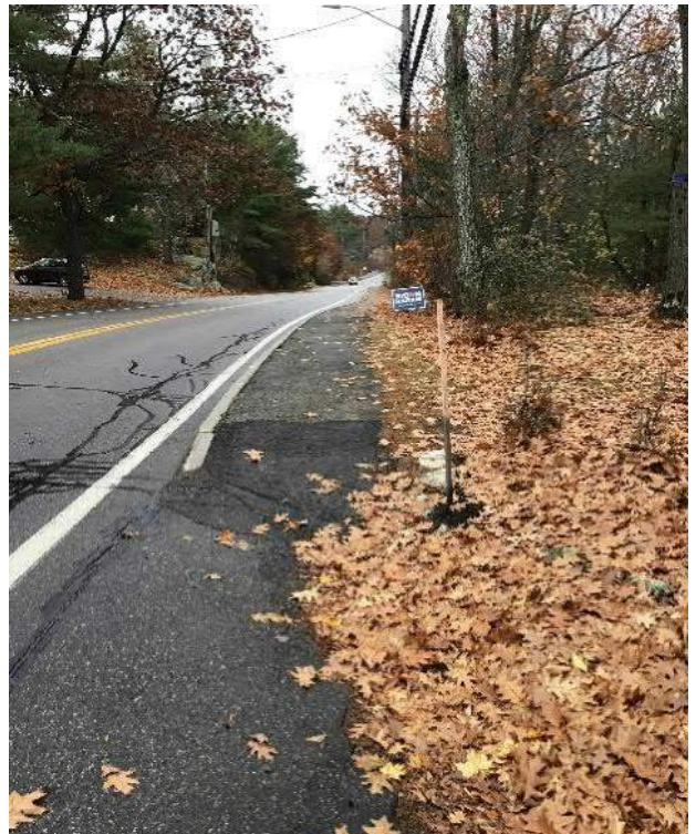
View of asphalt sidewalk and granite curb in the front yard crossing the proposed sewer, facing Southeast.
