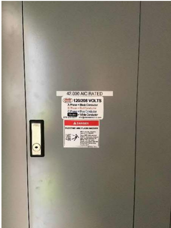
View of breaker box #1 exterior labels when closed.
