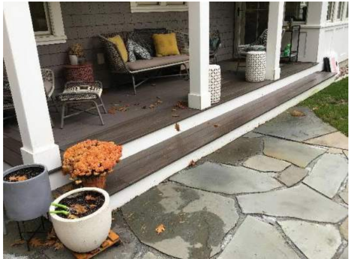
View of wooden deck and stone patio covering the approximate sewer lateral location, facing East.
