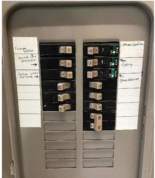
View of breaker box #2 circuit breakers and schedule adjacent to breaker switches.
