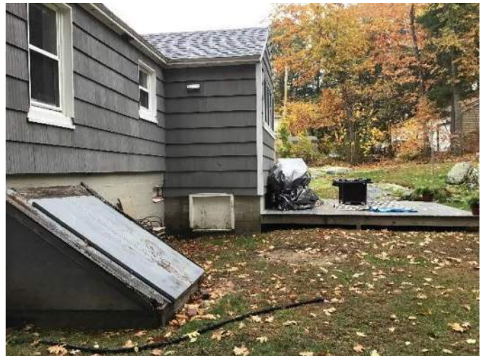
View of basement bulkhead and approximate septic tank location denoted by a patch of dirt.
