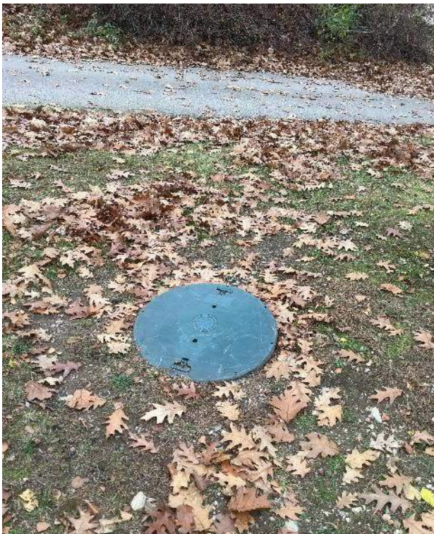
View of septic tank cap and tank located in the Northeast yard near the drive facing East.
