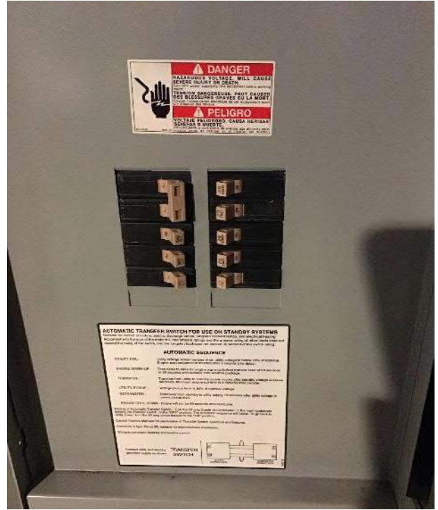
View of transfer switch front panel.
