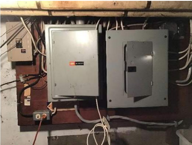
View of breaker boxes (#1 on left) and surrounding wall space in the basement, facing Southwest.
