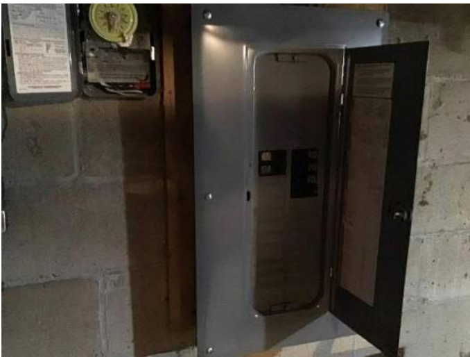
View of breaker box #2 panel and interior panel located in the basement.
