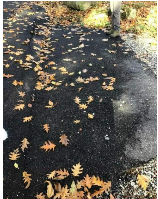
View of asphalt apron between Walker Bungalow Road and the gravel driveway facing Northwest.
