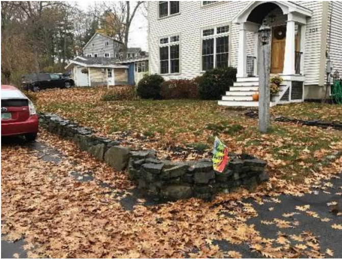
View of 201 Walker Bungalow Road front yard and small retaining wall facing Northwest.
