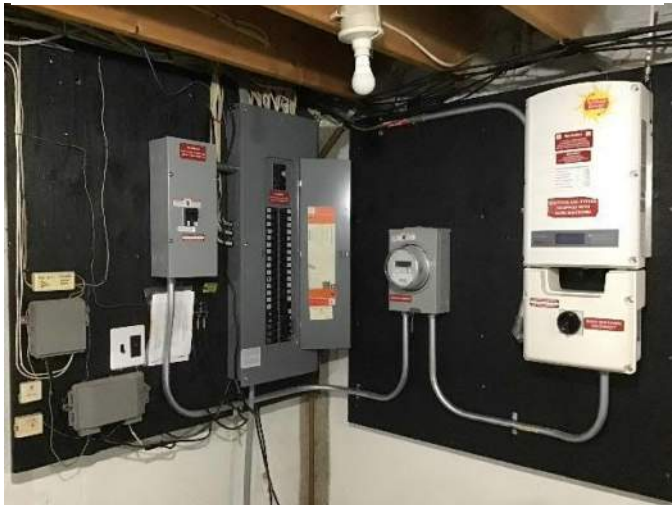
View of breaker boxes, solar power electrical system and surrounding wall space facing East.
