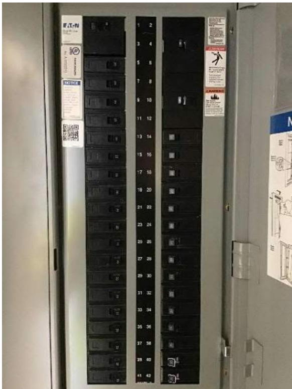
View of 200A breaker box #1 breaker panel.
