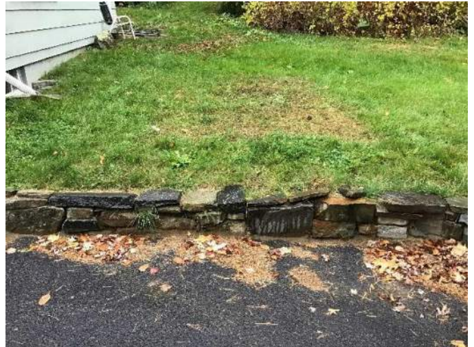
View of small retaining wall and location of the septic tank facing Northwest.
