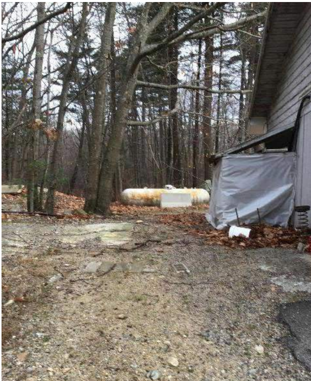
View of propane tank located in the woods behind the building facing Southeast.
