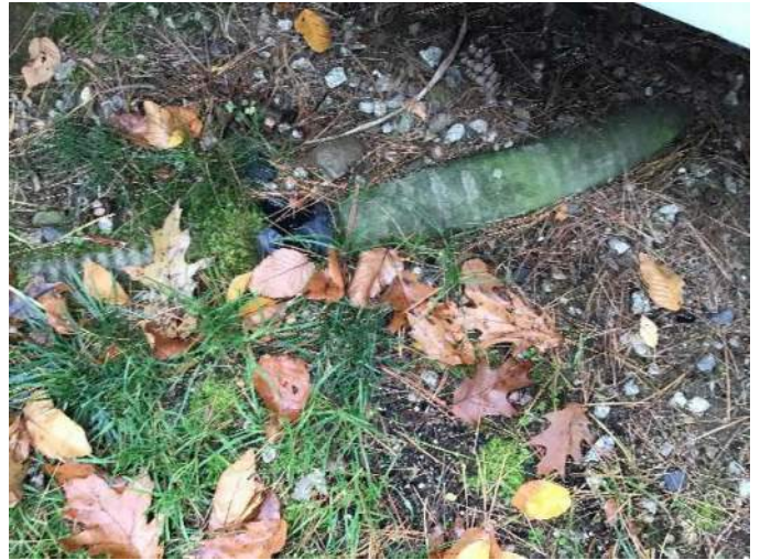
View of exposed sewer lateral located underneath the wooden deck facing Southwest.
