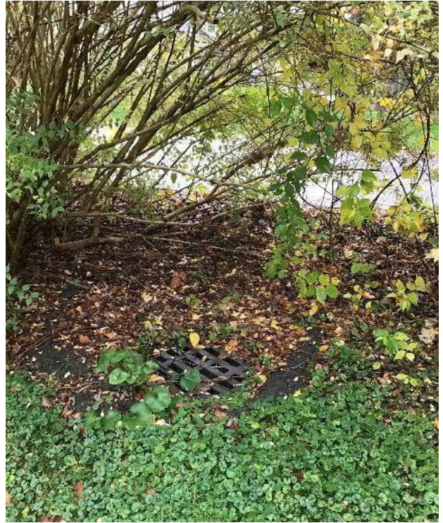
View of catch basin within the shrubs adjacent to the proposed sewer service path facing Southeast.
