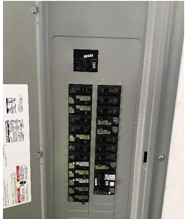
View of breaker box #1 (Siemens) circuit breakers.
