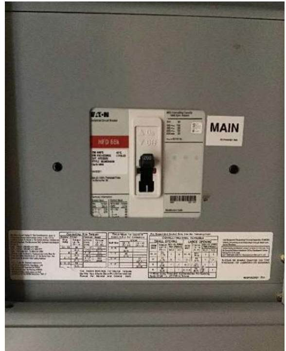
View of breaker box #2 (Eaton) 200A main breaker and model information.
