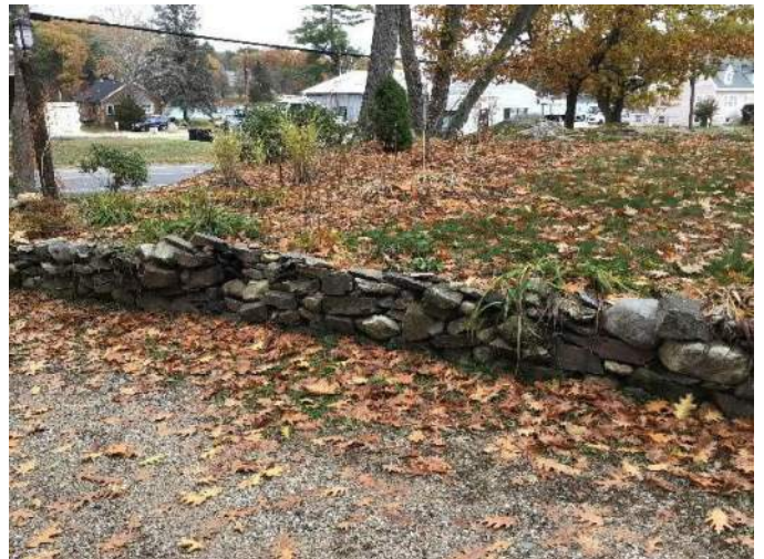
View of retaining wall along the East side of the driveway facing Northeast.
