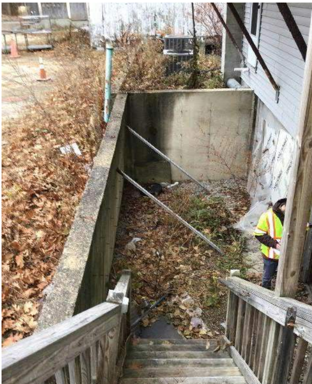
View concrete retaining wall and wooden steps to access the basement door facing Southeast.
