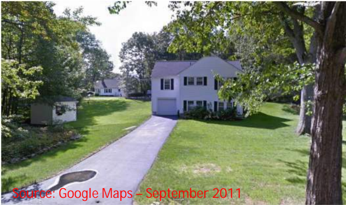
View of 131 Cliff Road from Walker Bungalow Road Avenue facing Southwest.
