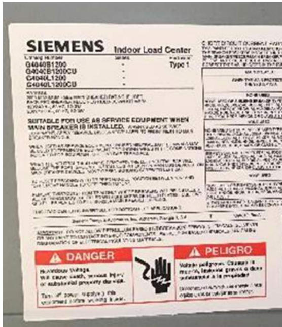
View of the breaker box model information and specifications.
